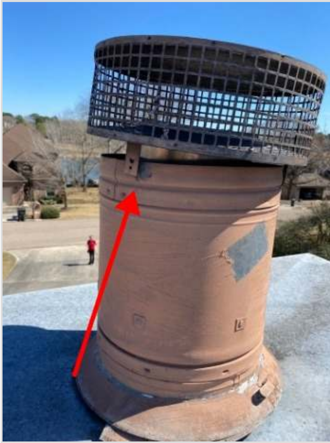
Sparker rest I'm not seated properly
