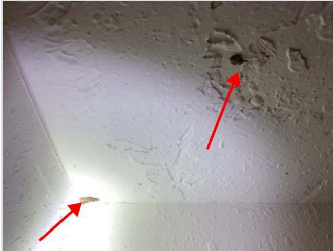
Possible wood destroying insects in the hall closet
