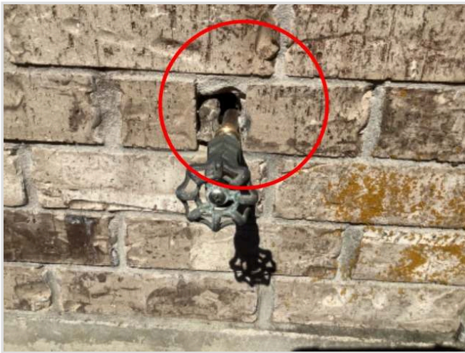
Area around faucet needs to be sealed to prevent intrusion of insects left side of house
