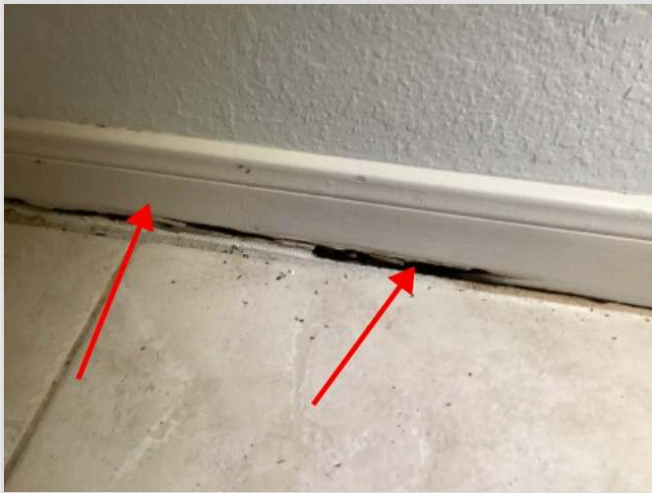
Trim board around flooring in kitchen is rotten. Recommend replacement
