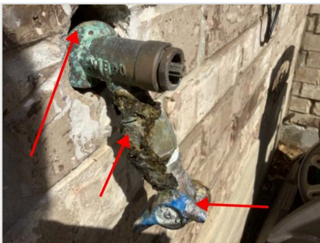
Area around faucet needs to be sealed to prevent intrusion of insects left side of house
