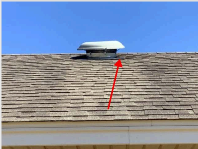
Flashing lifting on rear of house
