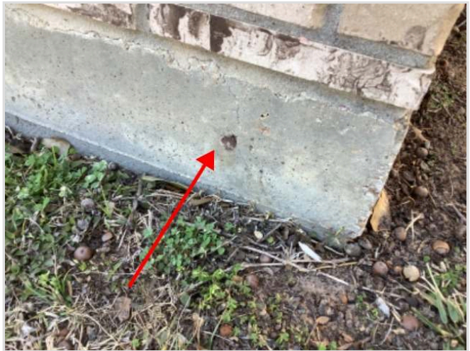
Exposed post tension cable right front of house
