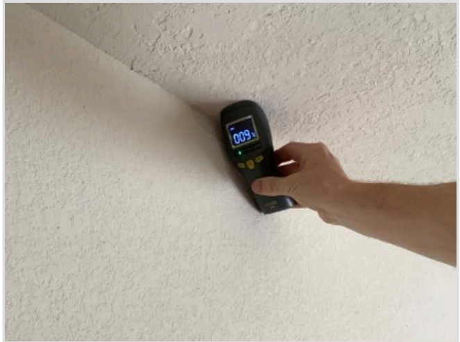
No current moisture noticed in ceiling
