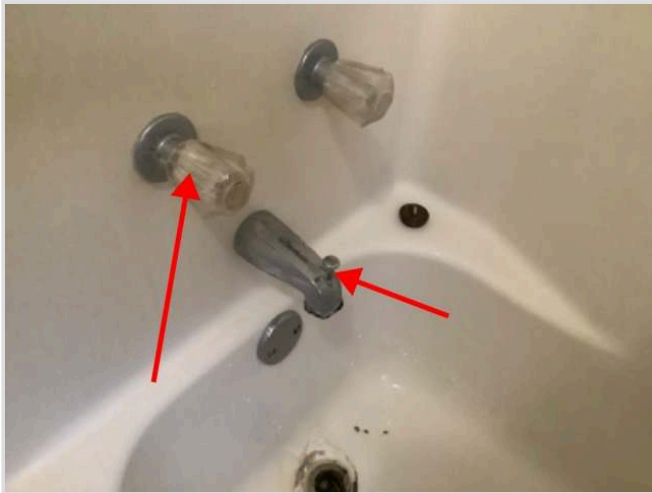
Hot water handle in master bathroom turns 360. Diverter on faucet is stuck and will not turn off
