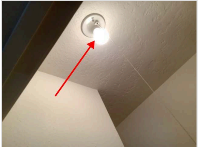
Unprotected lightbulb and secondary all
