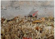
B. Grading and Drainage - Comments: Flat, Minor slope, High soil level in front right flower bed Down spout missing kick out at back left corner of house
