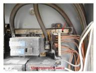
B. Branch Circuits, Connected Devices, and Fixtures Copper, No visible bonding of gas lines to ground
