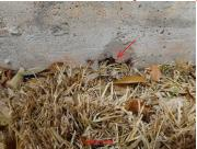
B. Grading and Drainage Flat, Minor slope, High soil level in front right flower bed Down spout missing kick out at back left corner of house
