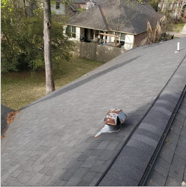
C. Item 3(Picture) Roof overview.
