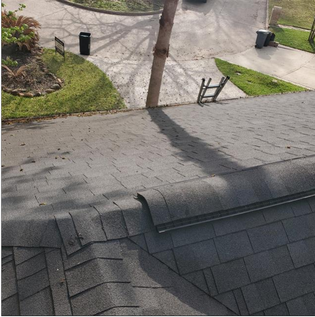
C. Item 1(Picture) Roof overview.
