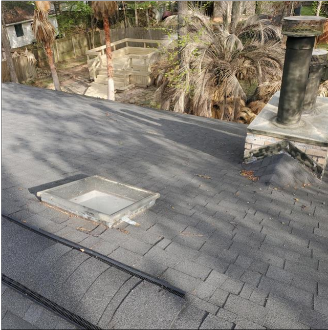
C. Item 2(Picture) Roof overview.
