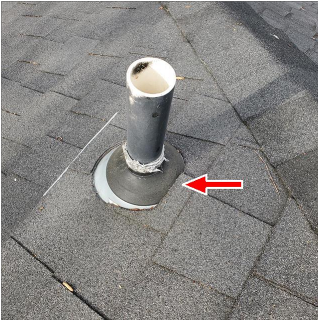
C. Item 6(Picture) Shingles should not be lifted over the back of the boots. The shingles should be cut around the boots.
