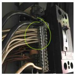
Anti-oxidant paste missing at main aluminum conductor terminals in distribution panel (see photo). Recommend having a qualified electrician apply paste as needed.
