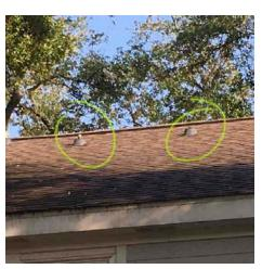
• Water has backed up under shingles due to debris on roof causing leak
