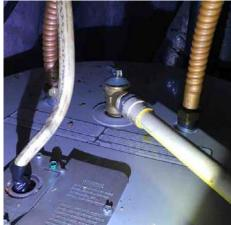
Rubber grument is not installed where electrical wire enters water heater wall
