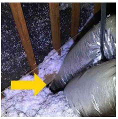
• Opening in fire barrier should be sealed with fire retardant caulk
