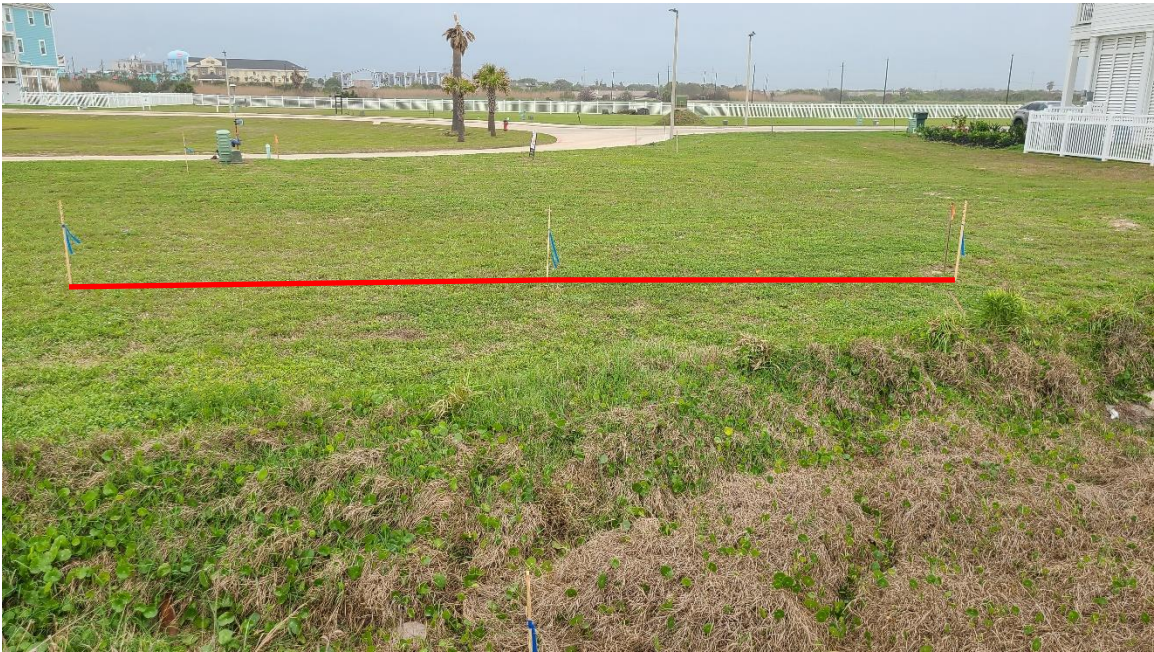
View of Lot 33 as seen from the dune. The 25' offset is shown as a red line.
