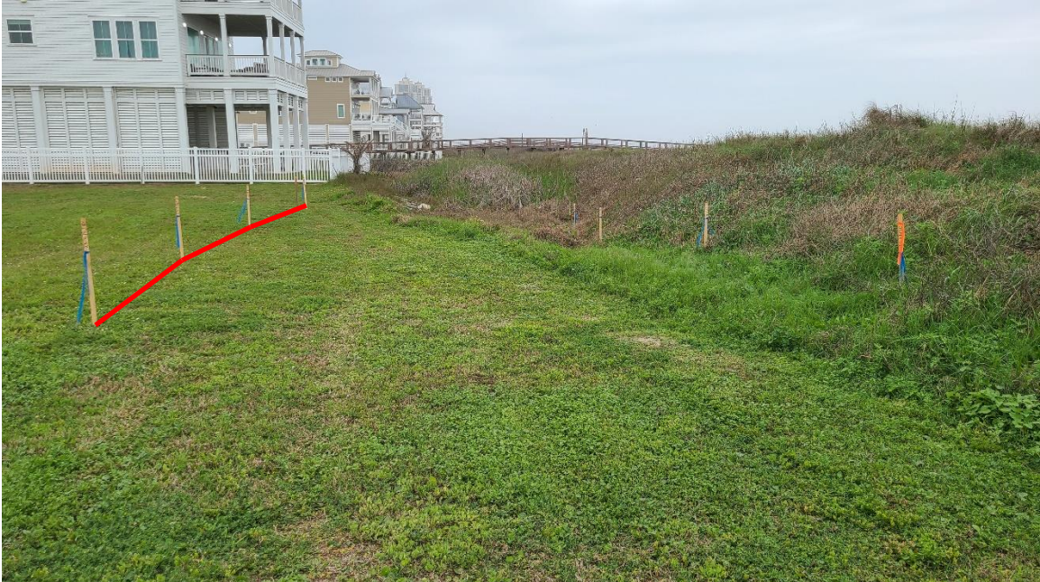
East view North Toe of Dune and 25' offset from North Toe of Dune. The 25' offset is shown as a red line.
