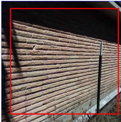
E. Item 7(Picture) Rear of garage
