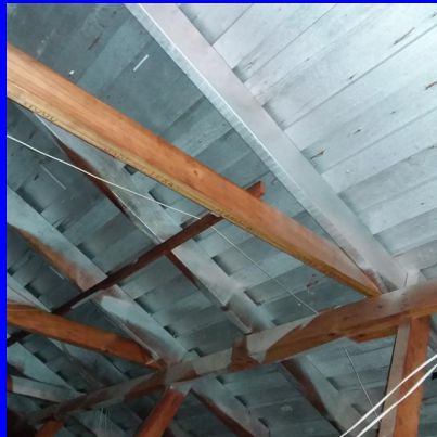
Roof structure stick built
