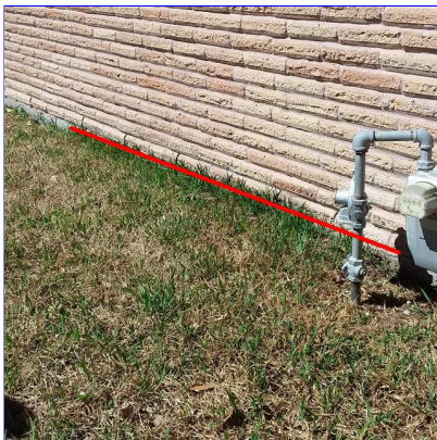
E. Item 5(Picture) Rear of home
