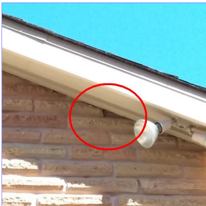
E. Item 11(Picture) Right side of home
