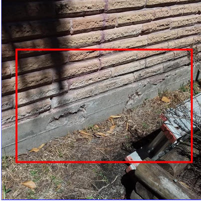
A. Item 1(Picture) Rear of garage
