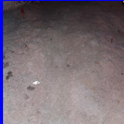
12 inches of blown insulation
