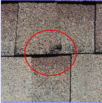
C. Item 2(Picture) Front left of home
