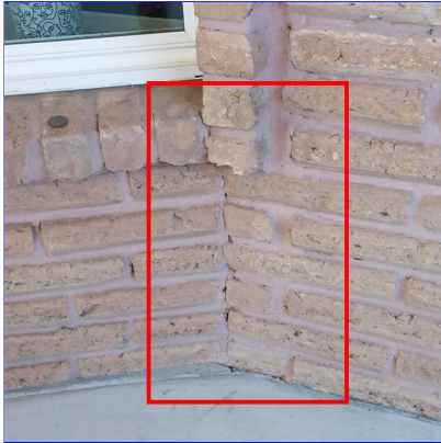
E. Item 1(Picture) Left rear of home (3/18/2021)
