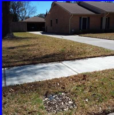
Water meter front left of home
