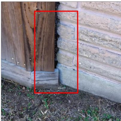
L. Item 3(Picture) Front left of garage
