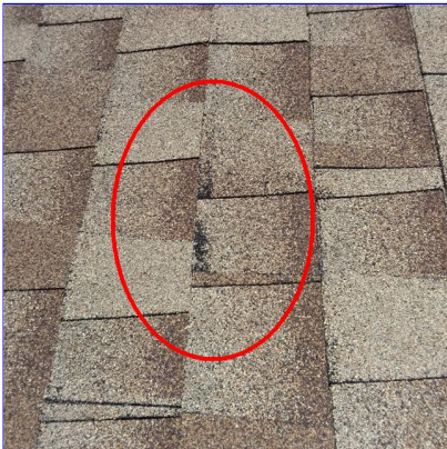
C. Item 1(Picture) Rear of home
