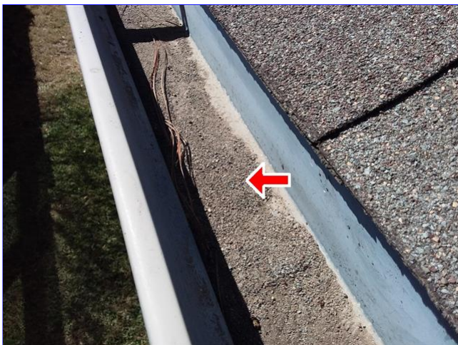
C. Item 1(Picture) shingle granule loss
