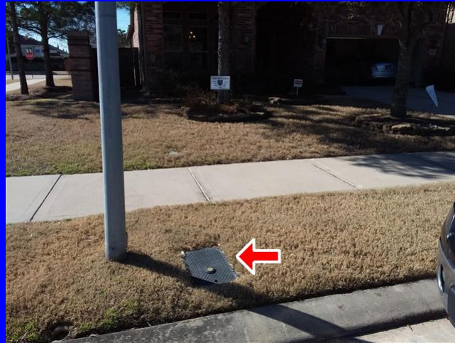
water meter location
