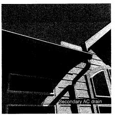
· Possible growth noted on the secondary drain line at the unit in the attic. This was only noted on the line and not on the unit itself FIX ED
