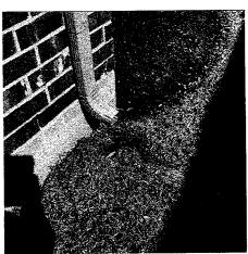
Please note, it is recommended to keep clearance of landscaping and grading 4-6 " below exterior siding. Areas of grading around the home appears to be above under 4-6" below the siding.
