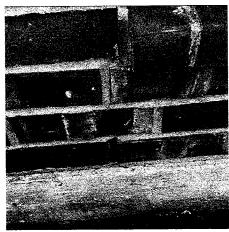
Lintel supports above doors and windows are starting to show signs of rusting. Rusting lintels can cause cracks in the brick due to the rust expanding over time. Recommend resealing lintels to avoid further damage.
