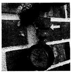
• Hose bib on East wall leaks at the stem seal when operated.
