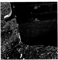
• Post tension cables are starting to show exposure in areas at the foundation. Recommend sealing these areas to prevent rusting / deterioration on the cables.
