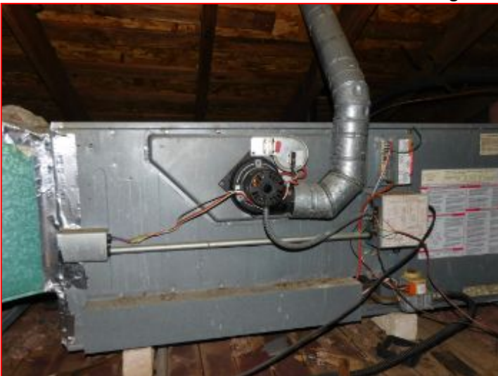
Furnace chimney is in contact or too close with the roof deck in the lower attic area. This area should have a minimum 1" clearance from combustibles and pass above the roof 2 ft" for safety reasons. There is evidence of roof deck overheating,
