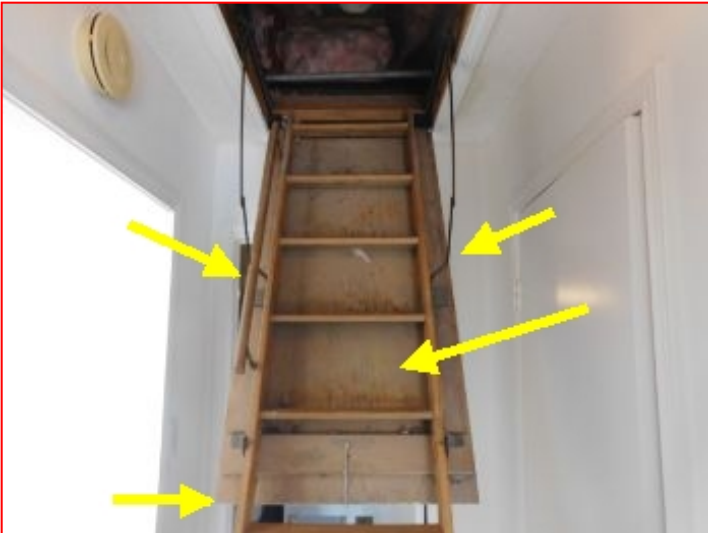
Insulate and weather-strip the pull down stairway door to promote insulation barrier to reduce moisture / condensation, Hot / Cold temperatures into the home from this area.
