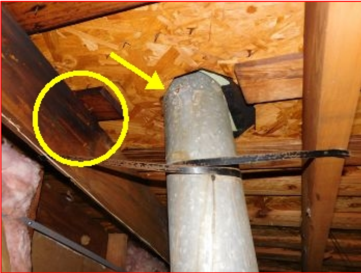
Furnace chimney is in contact or too close with the roof deck in the lower attic area. This area should have a minimum 1" clearance from combustibles and pass above the roof 2 ft" for safety reasons. There is evidence of roof deck overheating,
