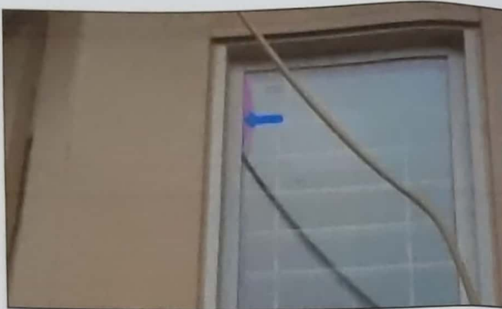
Window pane(s) that have lost their thermal seal. Signs of lost seals in the thermal pane windows may appear and disappear as temperature and humidity changes. Mainly at - Left side bay window
