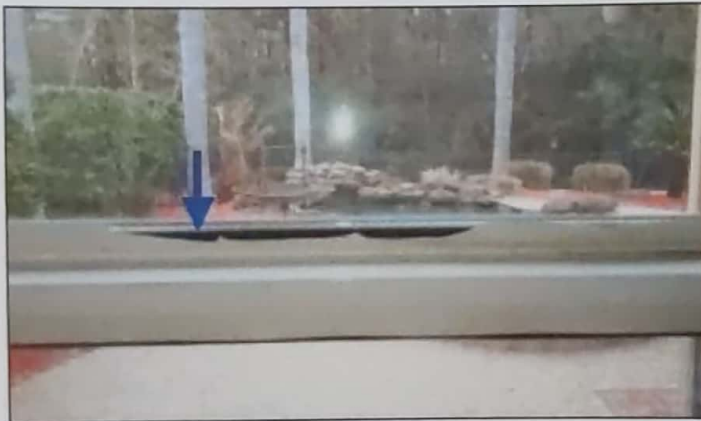
Glazing bead is damaged or deteriorated, recommend replaced or sealing to prevent moisture penetration. Mainly at - Breakfast nook
