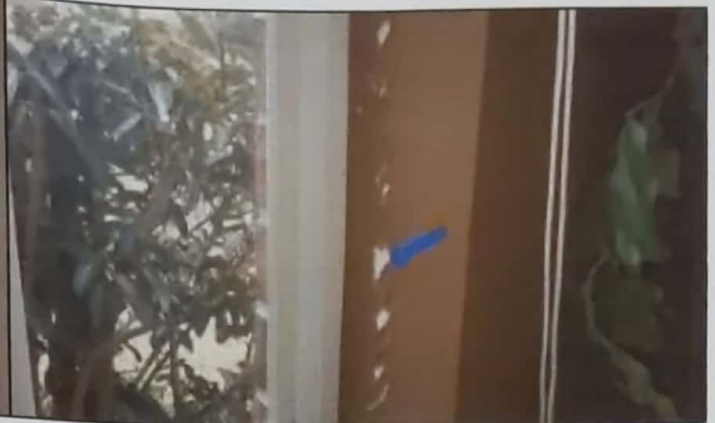
Sealant is needed around the interior of the windows between the window framing and the drywall to help prevent water penetration. Mainly at - Front left dining room
