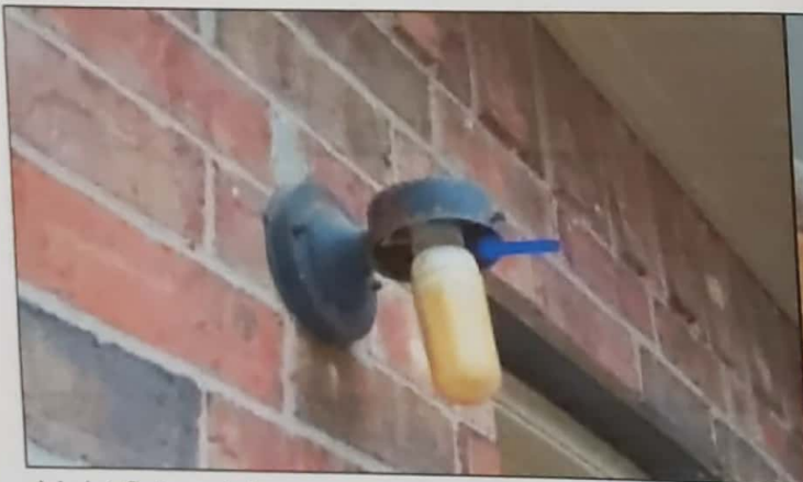
Light fixture(s) were missing their globe. Mainly at - Right side
