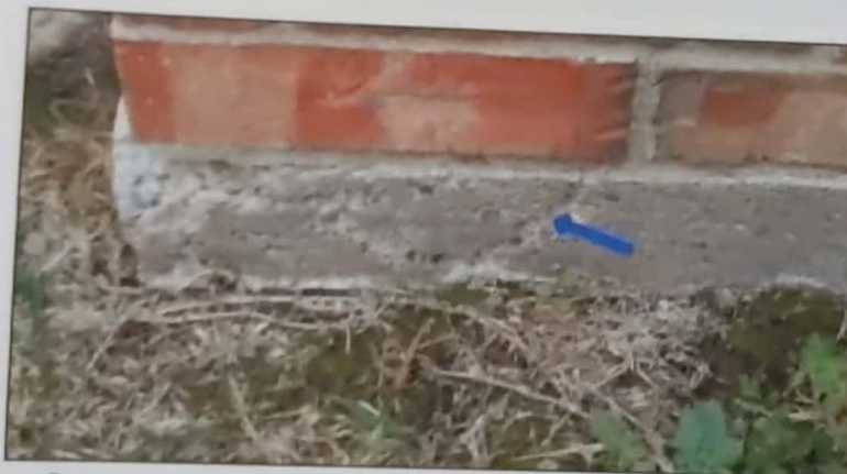
Corner pops were noted on the corner(s) of the foundation, these are usually considered cosmetic nature unless other movement is noted. Recommend sealing all cracks to help prevent further deterioration. Mainly at - Right side
