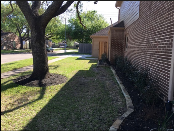
Trees were located within 15 feet of the foundation on the left side and front right corner of the home
