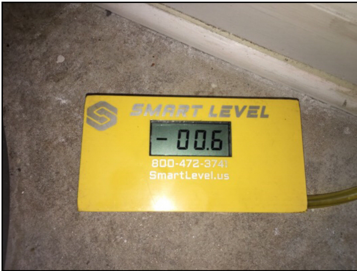
Foundation Elevation: Back left corner of home
