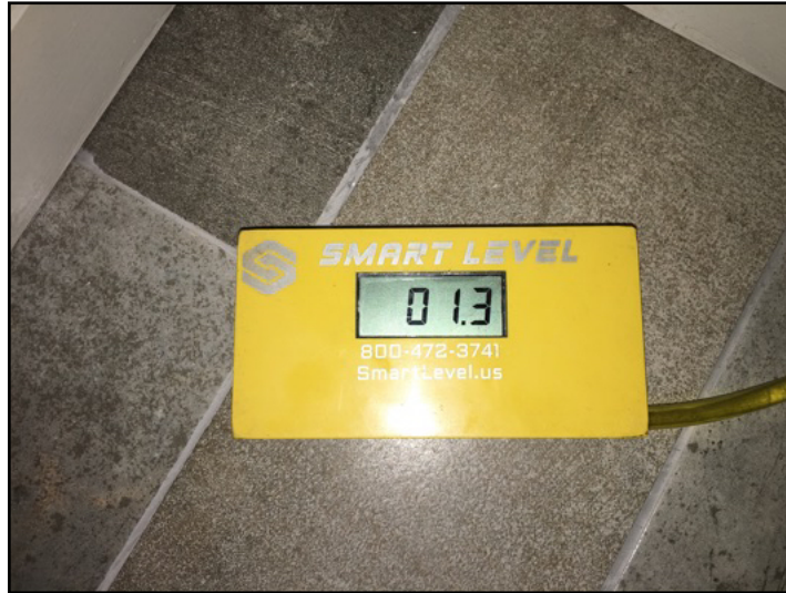
Foundation Elevation: Back right corner of home
