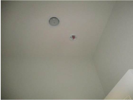
19. Missing smoke detector
