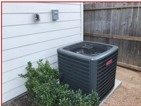
Ac overview, with shut off and outlet in place
