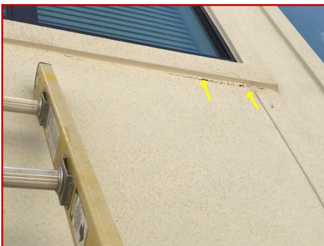
Cracked sealant
