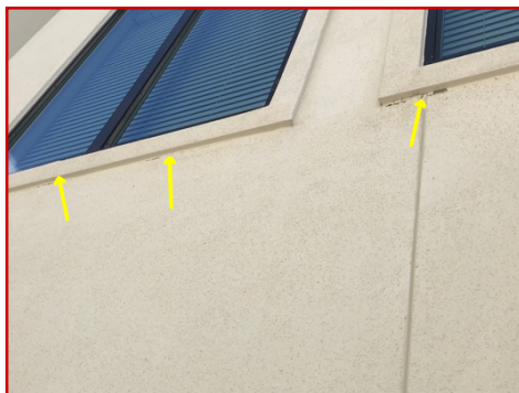
Cracked sealant
