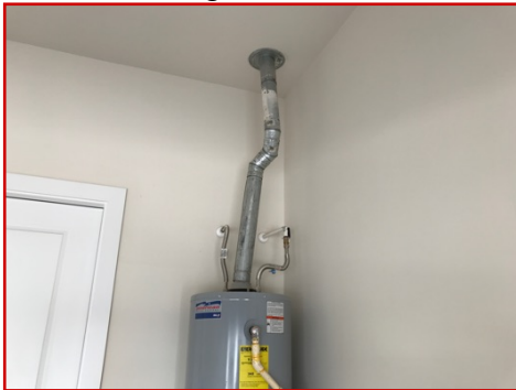
Appropriate water supply and venting
