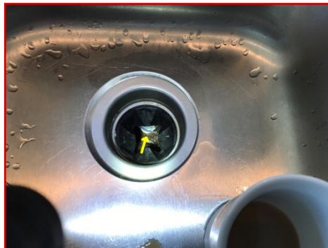
Foreign material in disposal
