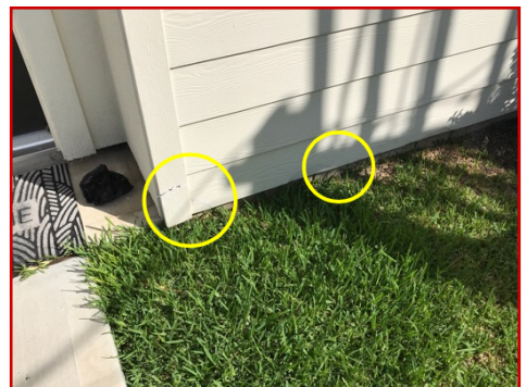
Damaged siding
