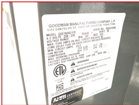
Goodman, 3.5 ton, charged with R-410A, max 40 amp breaker, mfg 2016
