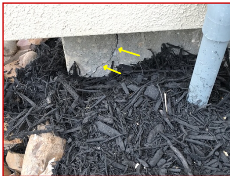
Corner crack
