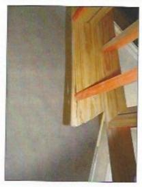
(3) Noted gaps in the insulation at the top of the attic stairs to the right. This may reduce the R value of the insulation system.
