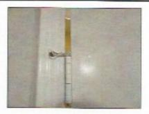
(2) Door stops are missing/need adjustment to prevent doors from hitting other interior components. Location(s): Multiple locations.
