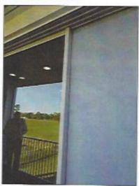
(4) Caulk/seal gaps at siding panels on the back side of the home at the second floor balcony.
