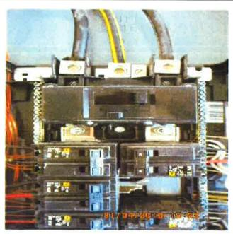
Oversized 40 amp. oven breaker(s) within the main distribution panel should be replaced. The purpose of the breaker is to provide protection to the conductors first and to the (6.8kW) appliance second. Over sizing is not allowed as the wires could overheat and or the appliance could burn without the breakers tripping.
