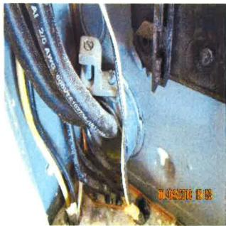
The main distribution panel and neutral bus bar do not appear to be properly bonded to ground.
