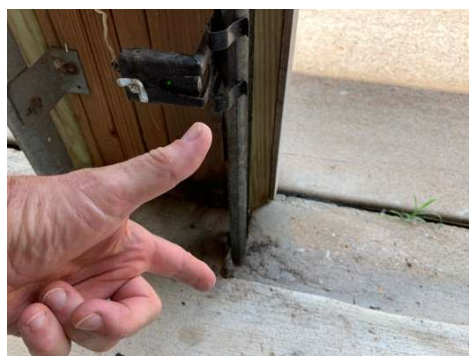
Photo eye sensor more than 6" off ground
