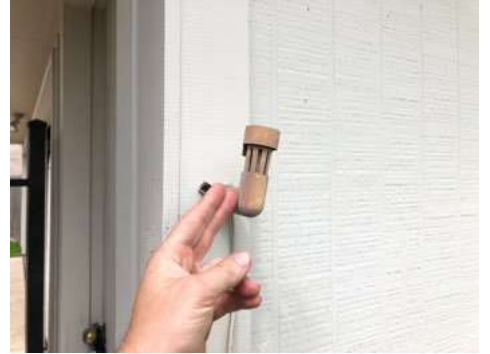
Garage right: rain sensor
