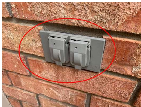
Exterior: Bubble cover recommended
