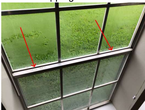
Windows Throughout house: missing hardware
