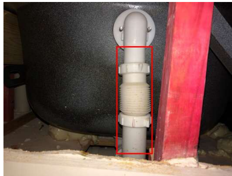
Bathroom 2: corrugated piping tub overflow drain
