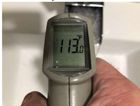
1st floor: Hot water temperature
