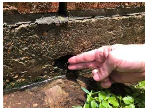
Right: exposed tendon head
