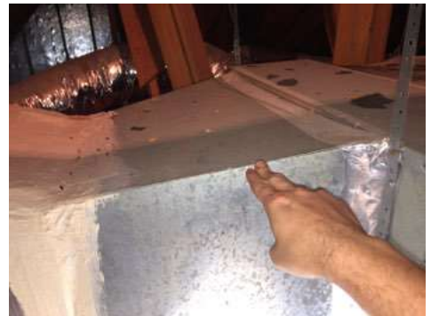
Unit 1: evaporator coils sealed
