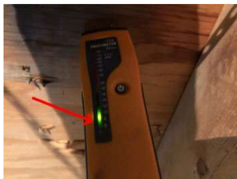
Moisture stains confirmed dry
