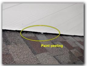
☑ 4. Missing step flashing where a roof intersects at exterior wall - Missing flashing will provide an opening for water intrusion and/or insect or rodent infestation
