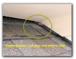
☑ 5. Lifting of roof shingle - potential area for water intrusion
