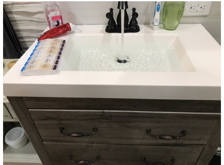
Typical view of testing drains at sinks
