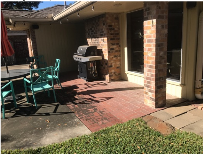
Rear patio deck obstructed view of slab
