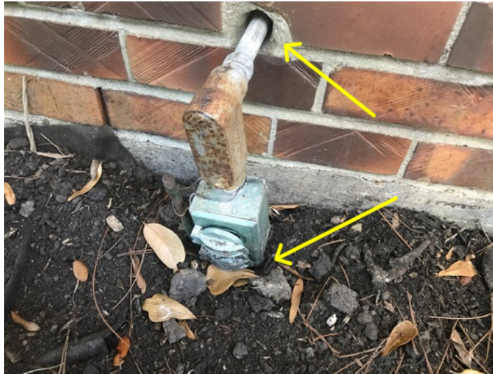
Outlet in contact with soil (front of house)
