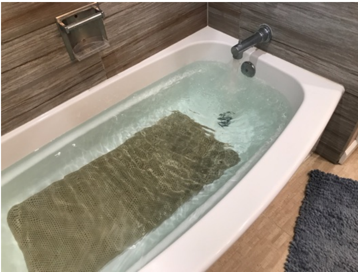
Typical view of testing drains at tubs
