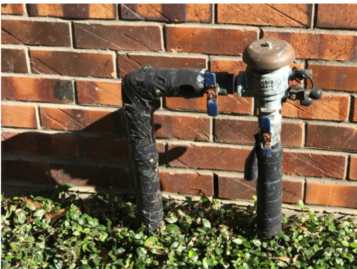
ICV at right side of house
