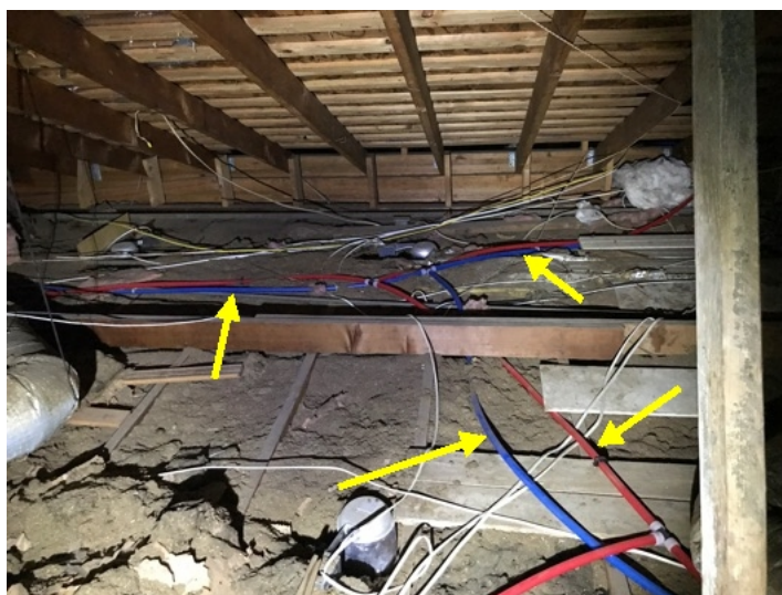
View of water lines in attic
