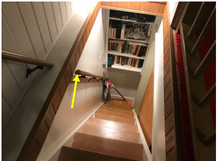
Open ended handrails
