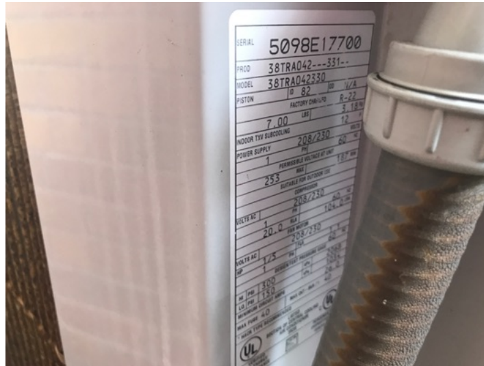
A/C condenser label: 1998 model, 3 1/2 tons
