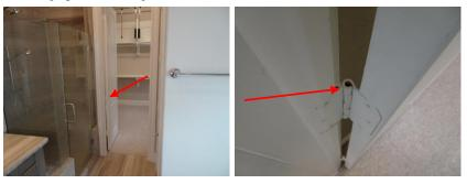
• The rubber seal is incomplete at the master bathroom shower stall door. The lower door seal is not contact the tile threshold. Repairs should be undertaken.
