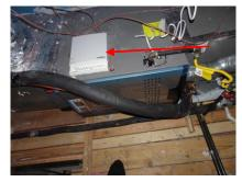
• The media air filter is not present in the attic. The heating and cooling system be cleaned and serviced.
