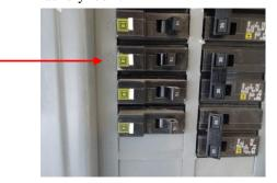
• The 20amp breakers in the electrical panel serving the garbage disposal and dishwasher are oversized (breaker #5 & #17). The wires (14AWG) routed to the breakers are only capable of handling 15amps. These breakers should be replaced with a 15 amp breakers.
