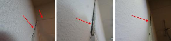
The under mount sinks are not adequately sealed at the countertops in all bathrooms.
