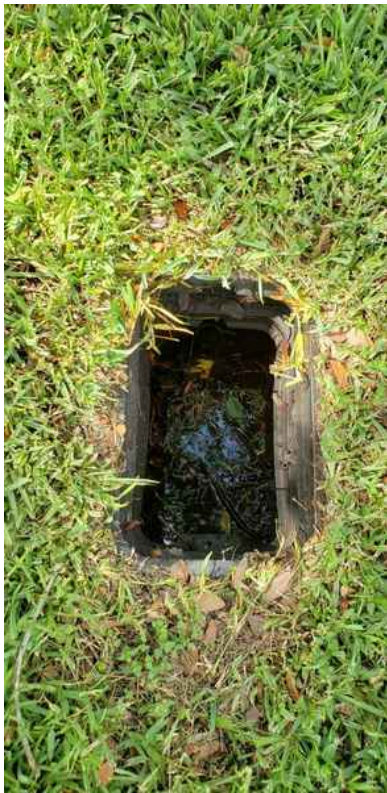
Material - Water Supply: Copper, PVC
