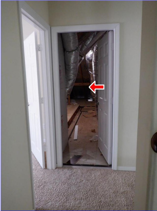
D. Upstairs back attic, Pulin support removed
