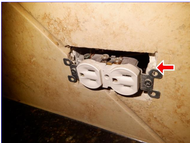
B. Kitchen back splash electrical outlety
