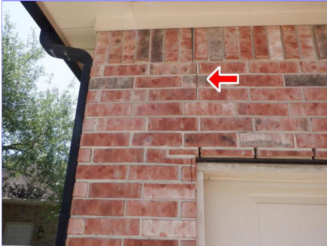
E. Front garage exterior wall
