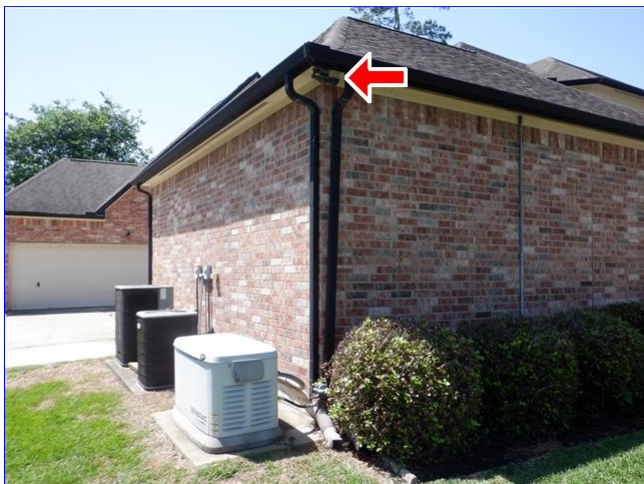
B. Back yard flood lights
