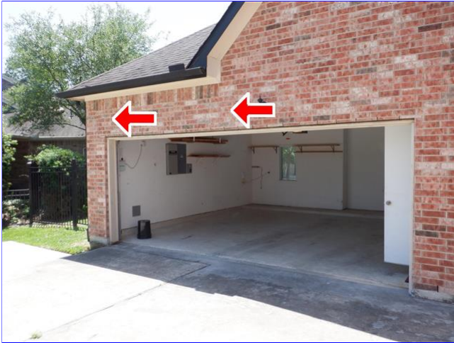
E. Front garage exterior wall
