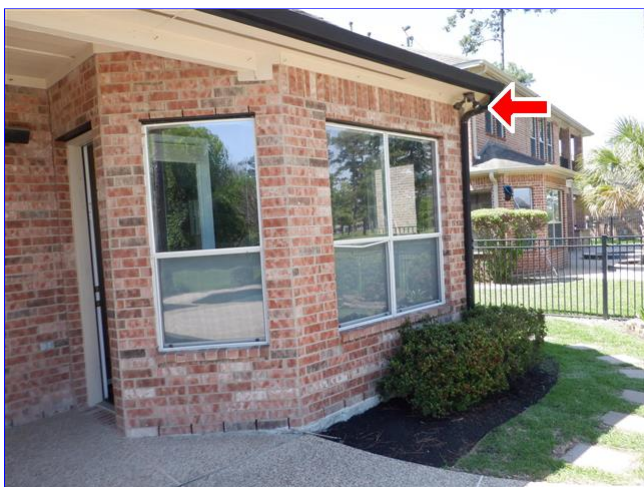
B. Back yard flood lights
