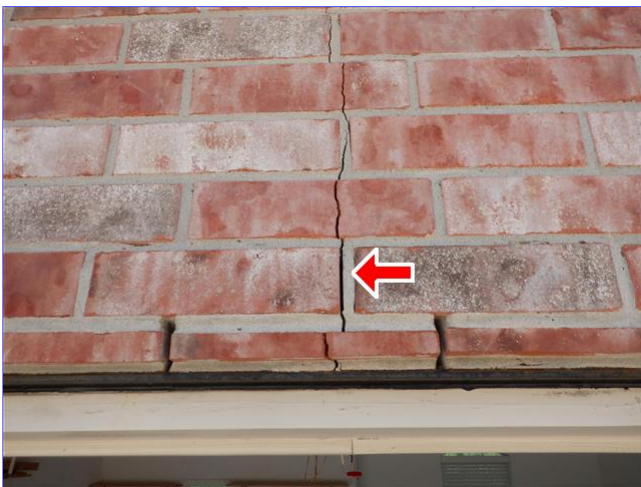
E. Front garage exterior wall
