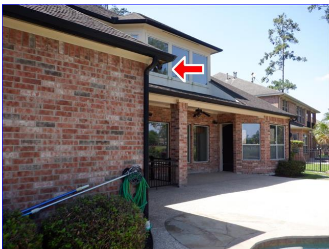
B. Back yard flood lights
