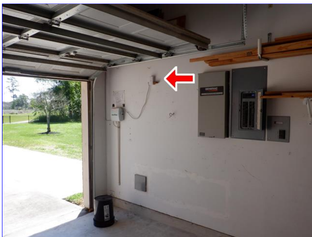
B. Garage electrical outlet
