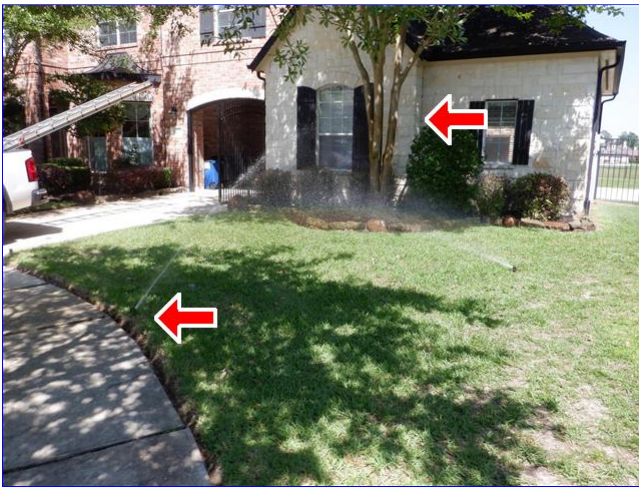
A. Zone 2, over spray on front of garage
