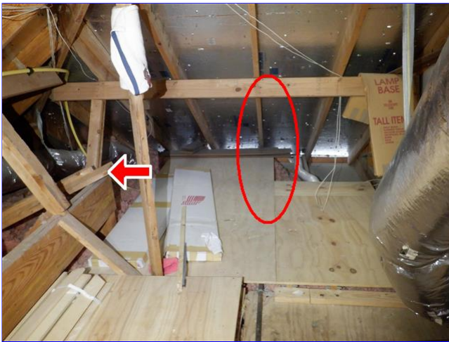
D. Pulin support removed
