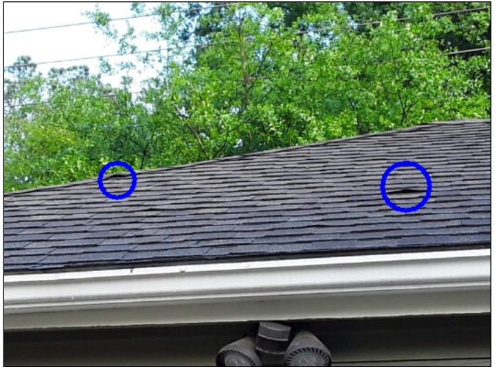
-Nails are noted backing out through the shingles, recommend repairs to help prevent shingles lifting during high wind conditions. Mainly at - garage
