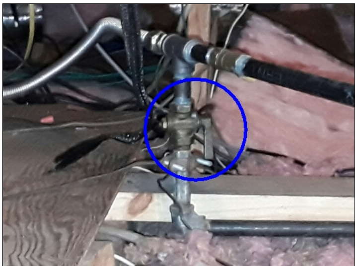
-There is an unapproved gas valve installed at the furnace unit.
