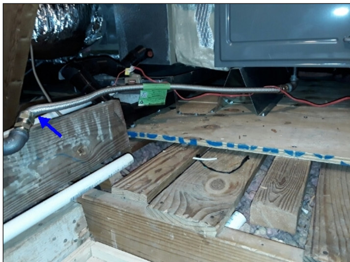
-There is no drip leg or sediment trap for gas lines on both furnaces. These helps prevent trash from clogging jets.
