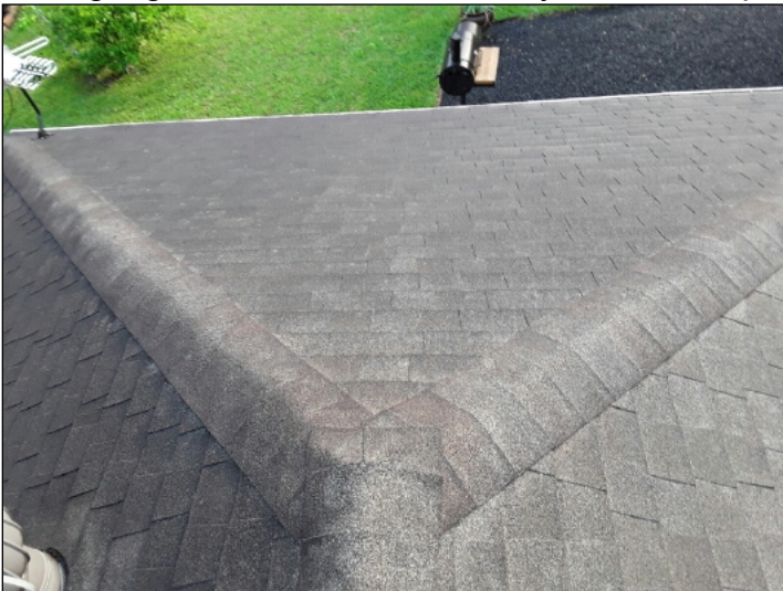
Overview of roof
