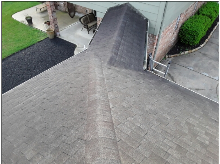
Overview of roof
