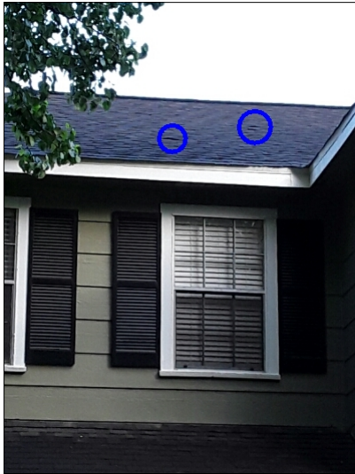
-Nails are noted backing out through the shingles, recommend repairs to help prevent shingles lifting during high wind conditions. Mainly at - front slope
