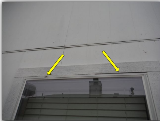
Missing header flashing over windows.
