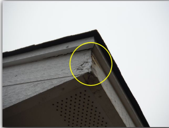
Fascia rot noted all along lower rear porch roof.
