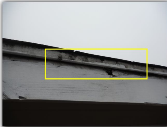
Fascia rot noted all along lower rear porch roof.
