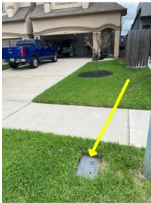
Water meter location
