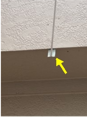
Trim piece is extending below the siding above and left of the front entrance door.
