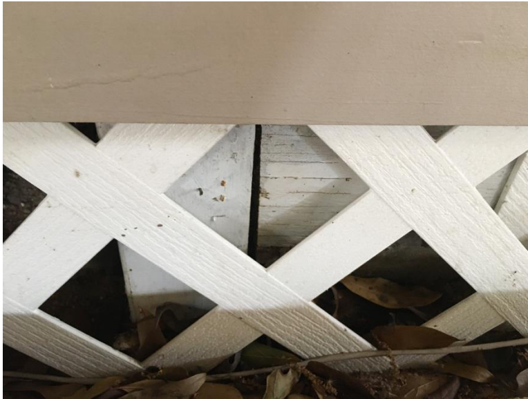
Wood to ground contact
