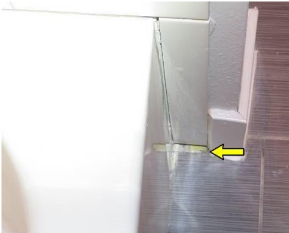
Example gap - upstairs Jack & Jill bathtub.
