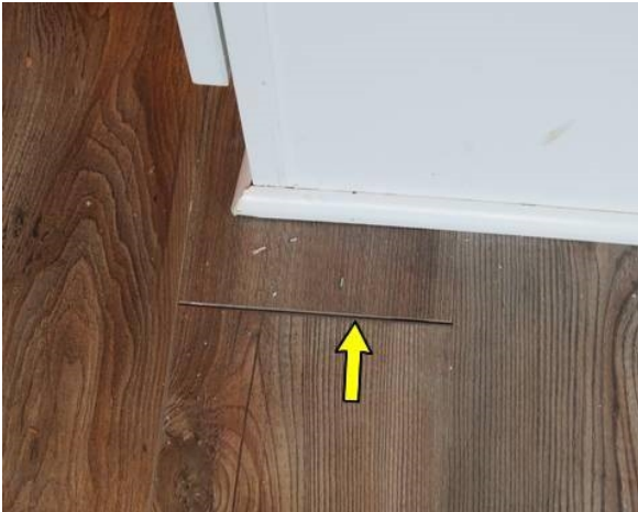
Example raised wood floor panel - near kitchen island.
