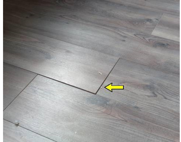
Example raised wood floor panel - breakfast area.
