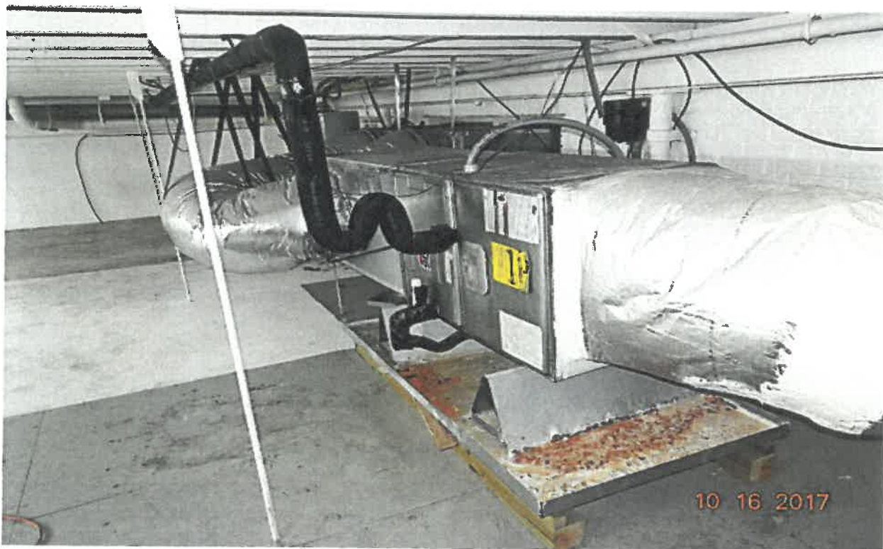
Photo # 10 HVAC unit on raised platform in garage
