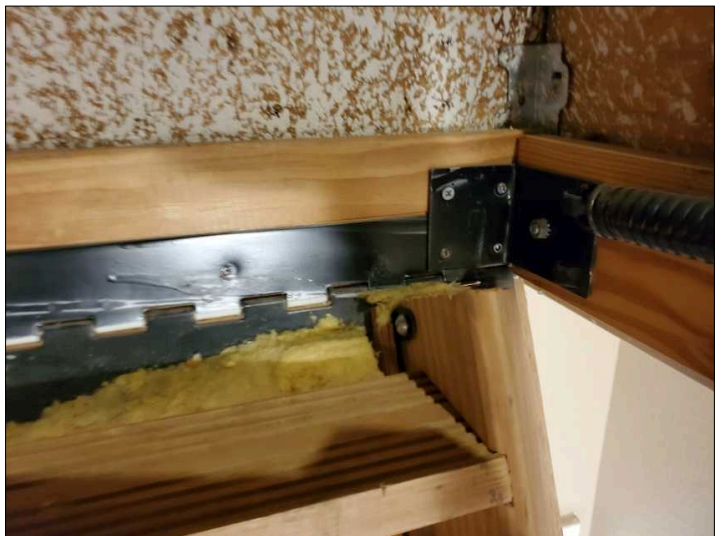
Ladder should be secured with 16d nails where indicated by manufacture, not screws.
