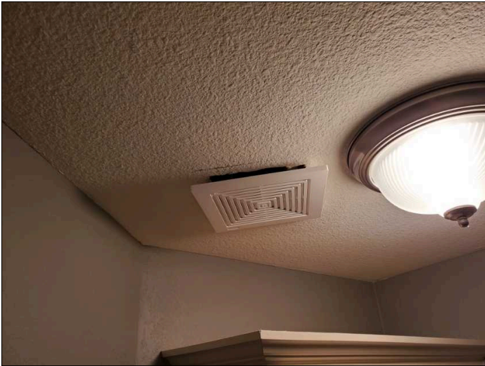
Loose exhaust vent fan.
