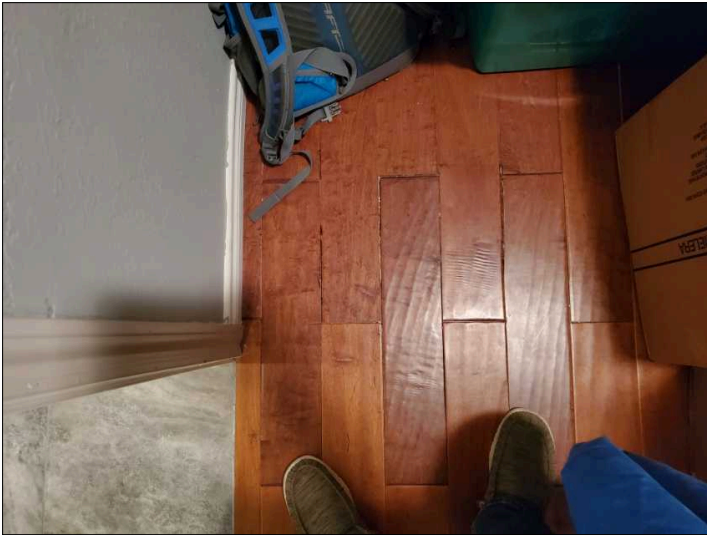
Poorly glued down floors in closet.
