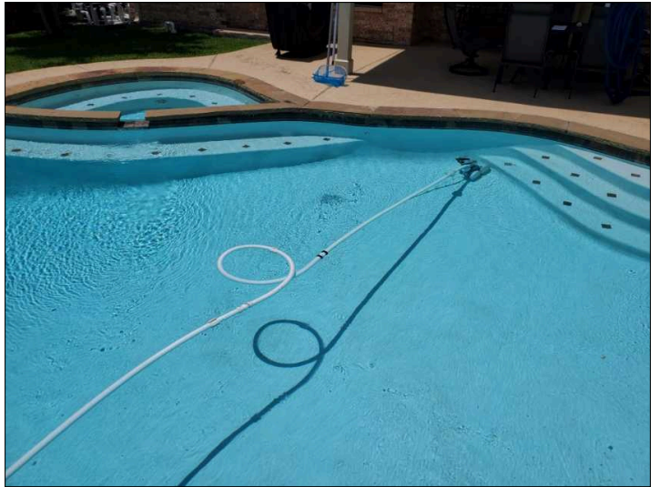
Leak noted in cleaner hose.
