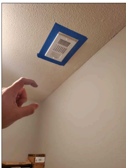
Some registers closed. These registers do not allow for air flow. No air flow can lead to mold growth and poor air quality in that location. Suggest opening and cleaning all registers.
