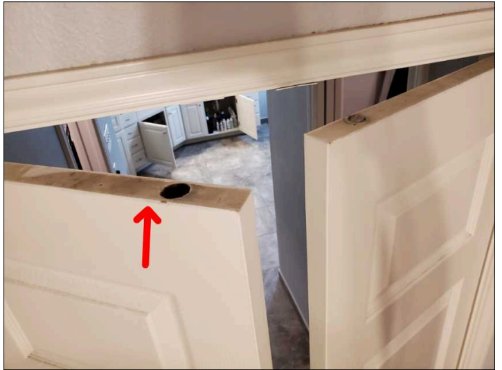
Doors not latching / shutting.
