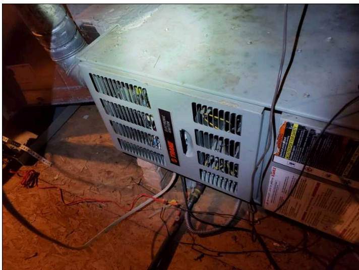
Furnace visually inspected and checked.
