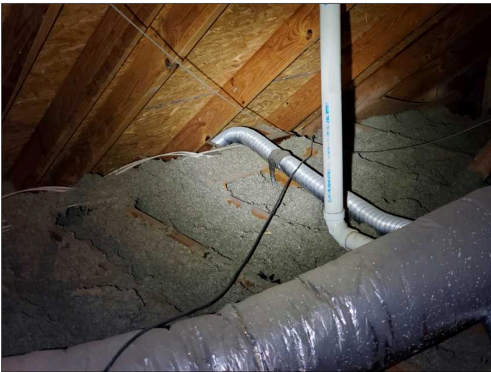
Loose exhaust vent fan.
