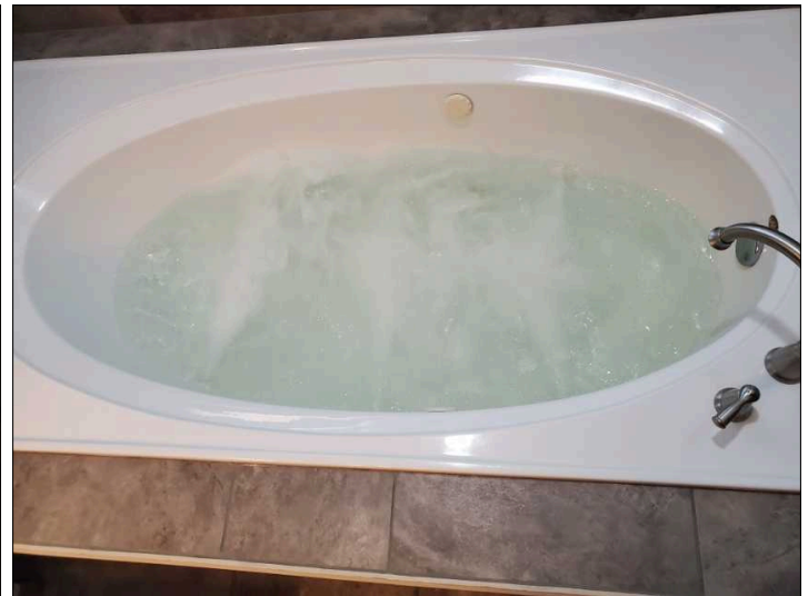
Operated. Timer and GFCI controlled.
