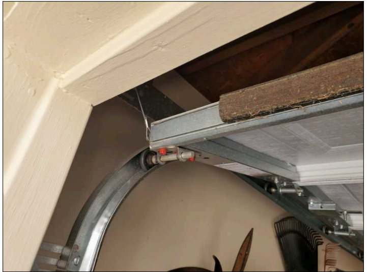
Floor seal is shorter than door.
