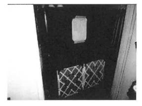
The heating and cooling for the condo was provided by a central supplied heated and chilled water system that provided conditioned water to a fan coil unit located in the foyer closet. The manufacturer of the equipment and age of the equipment was not determined at the time of the inspection; however the equipment appeared to be 20+ years old. (Information)
