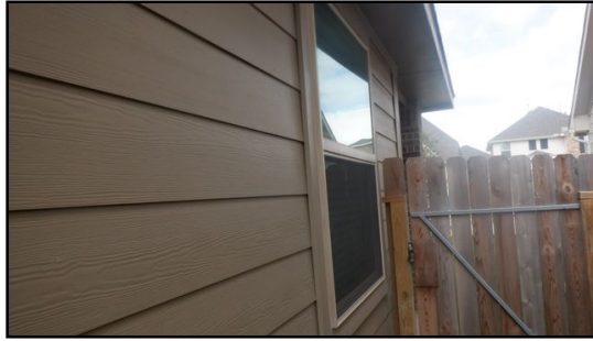
Cement siding is installed incorrectly.
