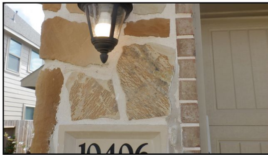
Observed minor grout separation around house number and stone above.
