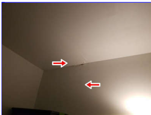
F. Item 4(Picture) garage
