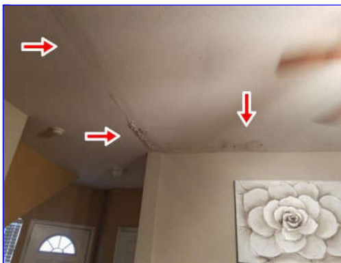
F. Item 5(Picture) living room
