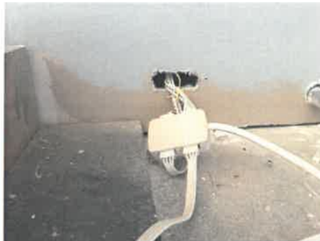
LED wire routing through the wall
