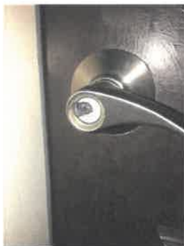
Damaged front door lock
