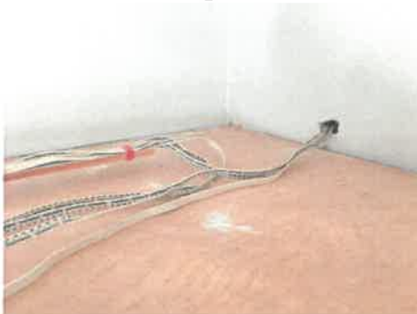
LED wire routing through the wall
