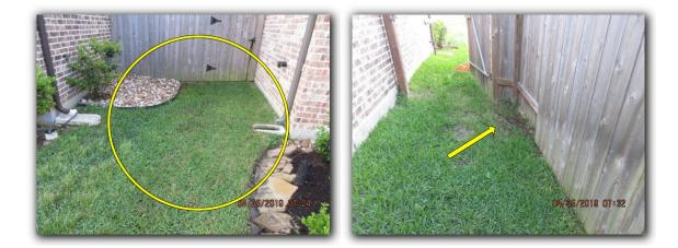
• Given the slope design of the finished grading, the protection from soil erosion appeared to be marginal at the time of inspection (Back Yard). The builder should be consulted to further evaluate this condition and remedies available for correction if needed.
