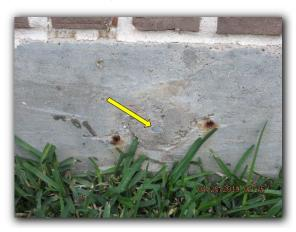
Surface deterioration (known as spalling) was observed along the perimeter beam of the foundation.
