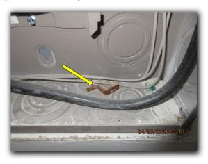
The metal bushing where the service conductors enter through the box is not bonded. Current building standards require bonding metal bushings where the service conductors enter through concentric knockouts.
