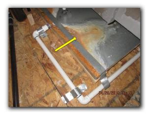
• The openings in the evaporator coil cabinet where the refrigerant/drain lines enter/terminate should be sealed properly to reduce the risk of air leaks.
