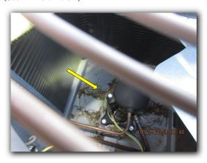
• Debris was noted in the safety pan installed below the evaporator cabinet. The pan should be emptied and cleaned to provide adequate drainage in the event of water accumulation.
