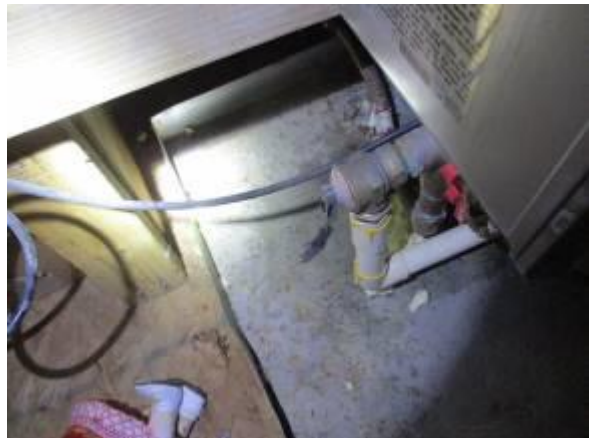
Active dripping at the roof jack/Standing water in the water heater pan
