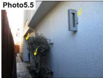
Penetration Sealants/ Seal
