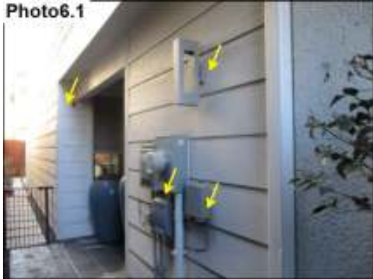
Penetration Sealants/ Seal
