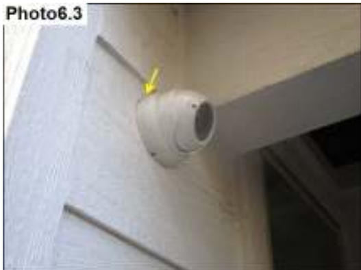
Penetration Sealants/ Seal
