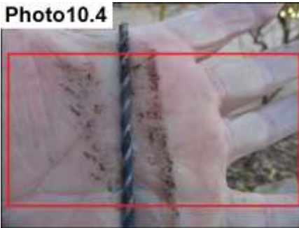
Confirmed Substrate Damage/ Repair And Add Relief
