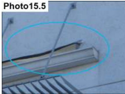
Scupper Flashing Sealants/s Seal
