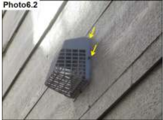
Penetration Sealants/ Seal
