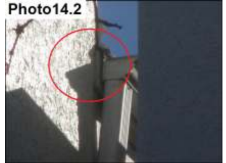
Roof Diverter Flashing Sealants/ Seal
