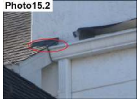
Roof Diverter Flashing Sealants/s Seal
