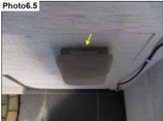
Penetration Sealants/ Seal
