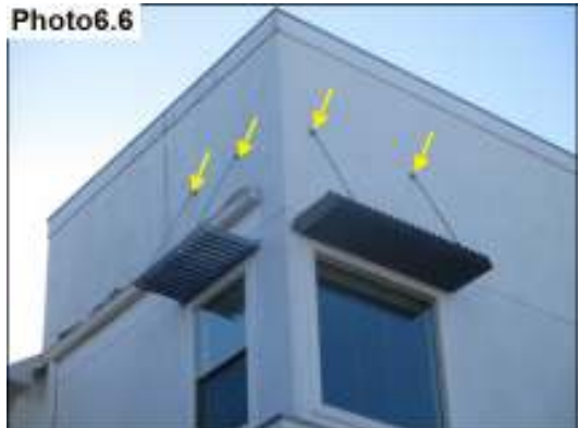
Penetration Sealants/ Seal
