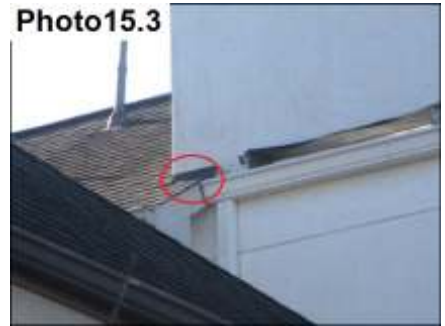
Roof Diverter Flashing Sealants/s Seal
