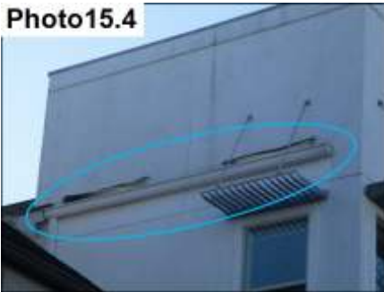
Scupper Flashing Sealants/s Seal
