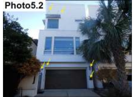
Penetration Sealants/ Seal
