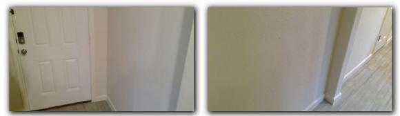
Evidence of previous repairs observed in interior walls at one or more locations. It appeared to the inspector that the sheetrock repair was due to previous flooding of the house. The sheetrock repairs did not appear to be performed in a usual and customary building practice manner. Seams were very noticeable.
