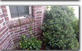
Weep holes had been closed at some locations and other mortar was removed higher up with what appeared to be an attempt at weepholes or drying out of the walls due to previous flooding of the house. The removed mortar should be patched and the lower weepholes need to be opened to properly maintain the moisture barrier drainage system in the exterior wall system.
