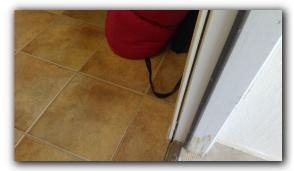
$\blacksquare$  Damaged weather stripping observed at one or more exterior door locations
