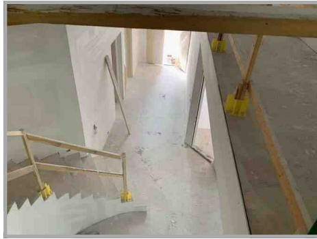
Entrance from 2nd floor
