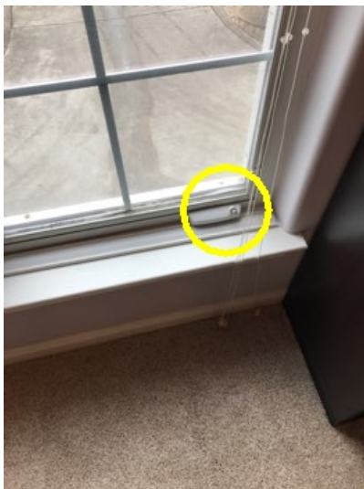
The right side front bedroom window is missing its hand crank.
