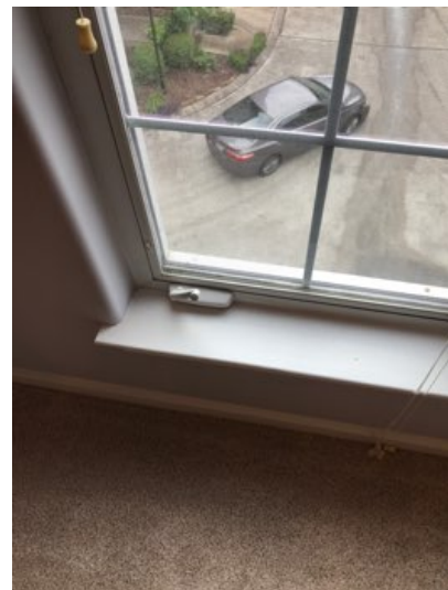
The right side front bedroom window is missing its hand crank.
