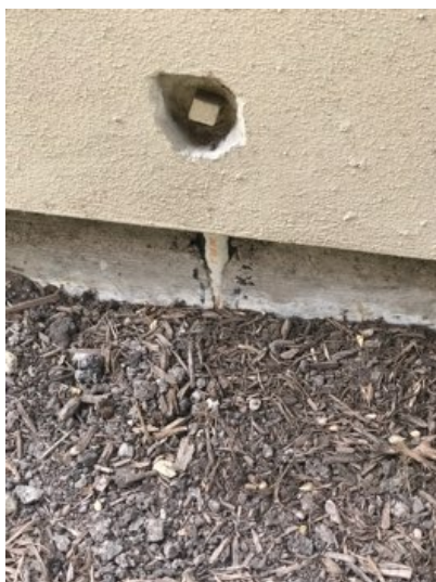
Drain cleanout was observed at the right side of the home.
