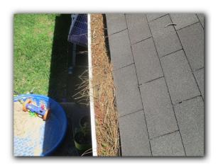
Recommend installing splashblocks or leaders under gutter downspouts to divert the runoff at least 2 feet away from the foundation.
