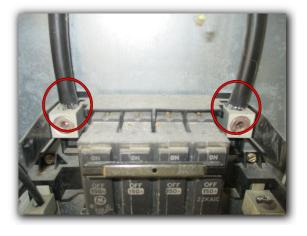
There is a white wire used as a hot conductor connected to the breaker for the A/C system. Normally the white wires are neutral. When used as a hot conductor, the white wires
