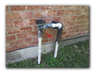
The anti-siphon valve for the sprinkler system has froze and broke. As a result, the sprinkler system could not be tested.
