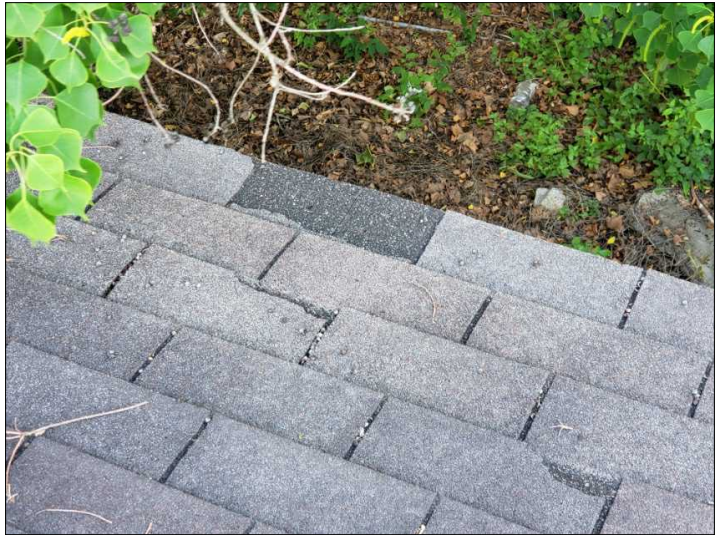
-There are damaged or missing shingles on the roof, recommend repairs or replacement of damaged shingles.
