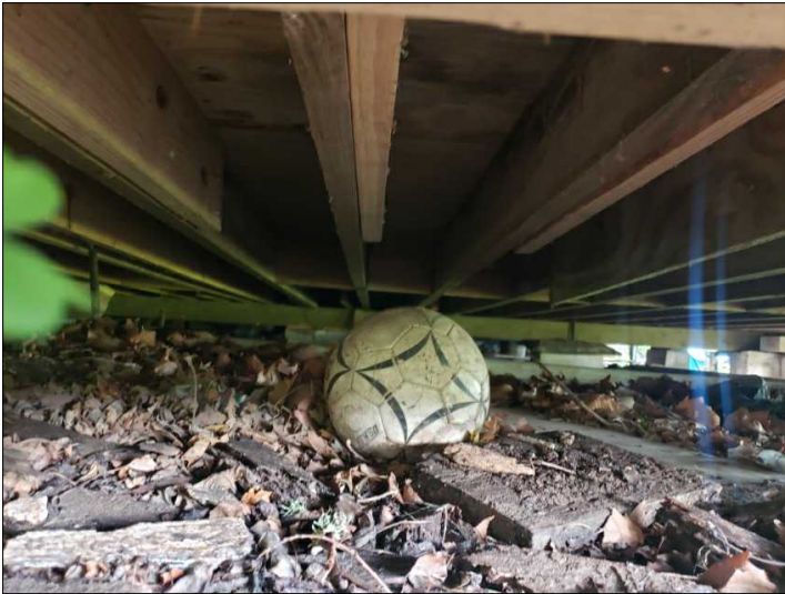
Overview of crawlspace.
