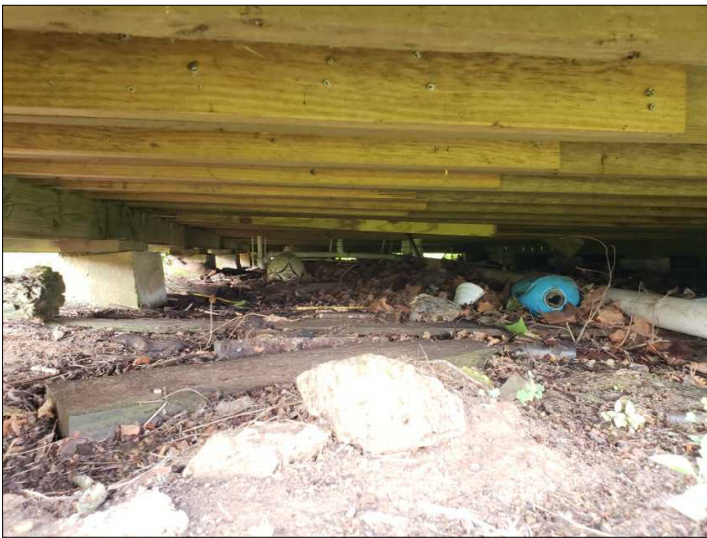
Overview of crawlspace.
