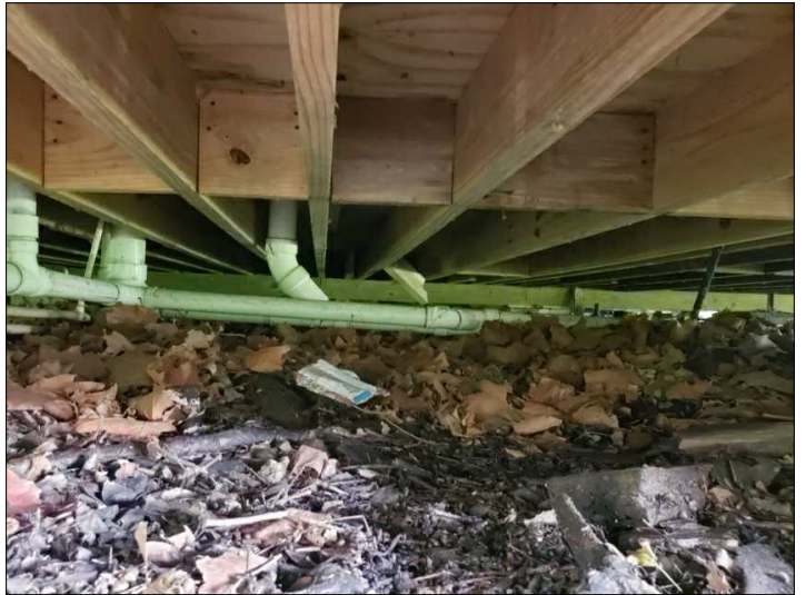
Overview of crawlspace.
