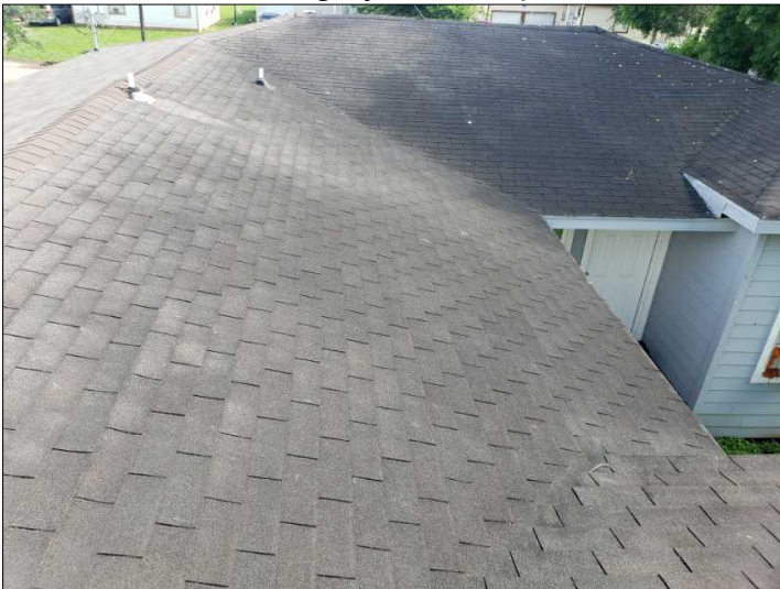
Overview of roof
