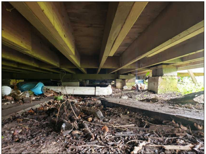
Overview of crawlspace.
