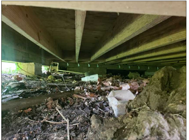
Overview of crawlspace.
