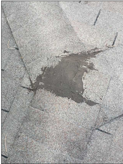
-Signs of improper previous repairs were noted on the roof. Recommend a roofing professional verify the integrity of the repair.
