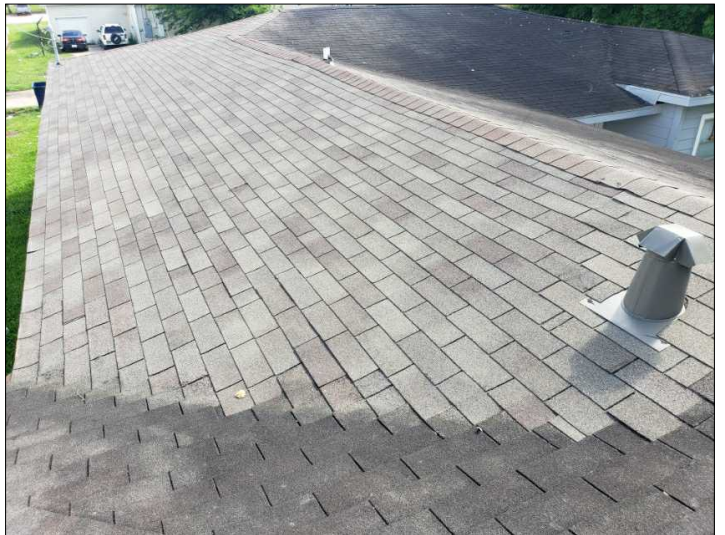
Overview of roof
