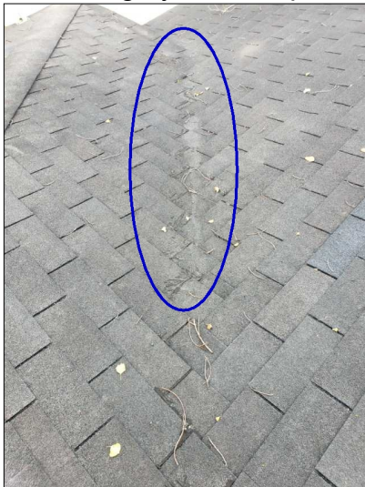
-Signs of improper previous repairs were noted on the roof. Recommend a roofing professional verify the integrity of the repair.
