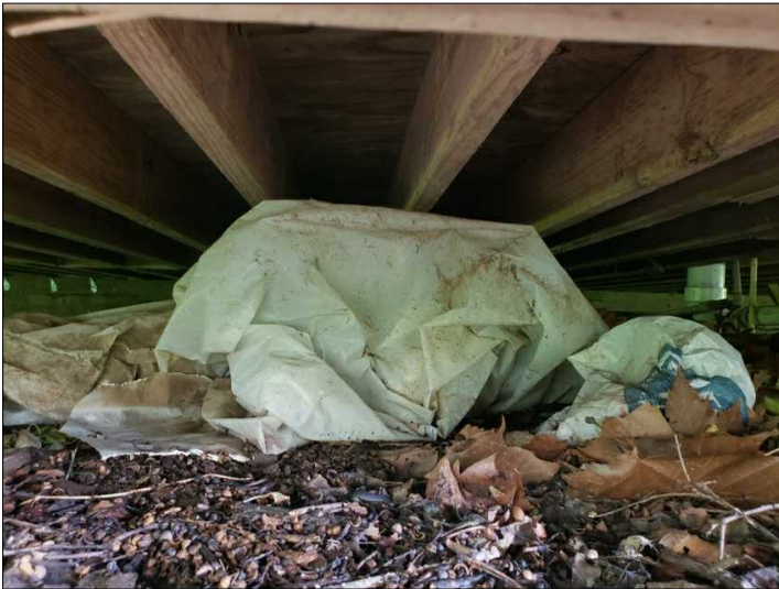
Overview of crawlspace.
