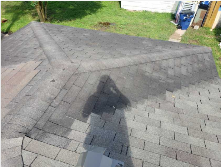
Overview of roof
