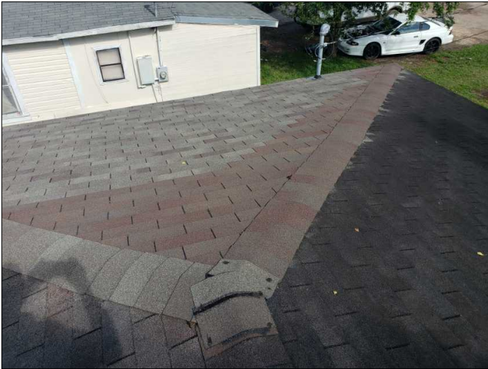
Overview of roof
