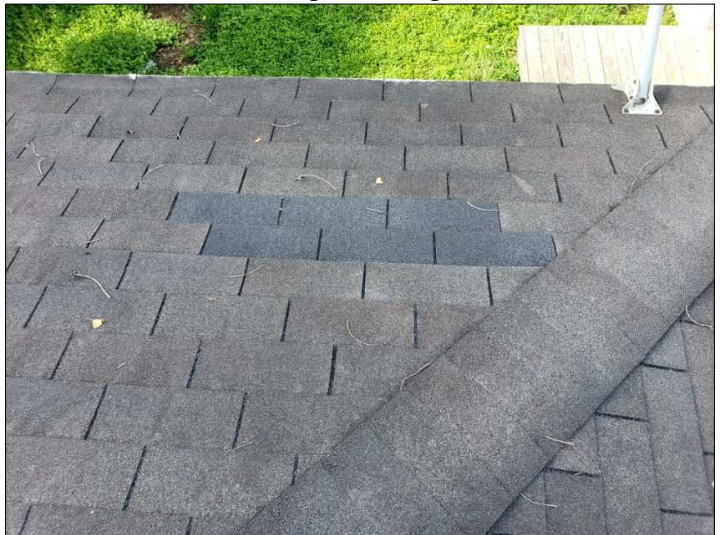
-Signs of previous repairs were noted on the roof. Indications are that they are working as intended at time of inspection.
