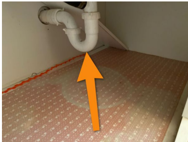
2nd Floor Hall Bathroom
