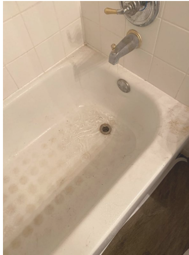
2nd Floor Hall Bathroom
