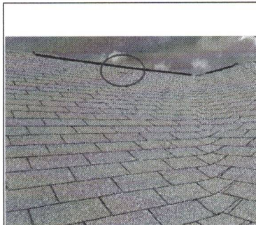
Southeast corner, minor lifted shingle
