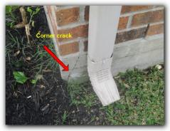
**Note:** The grade beam surface has had an application of dry patch sometimes called slab dressing applied typically to mask deficiencies in the finish. The application effectively conceals the beam surface from view and may conceal cracks, defects etc in the foundation as well as insect entry
