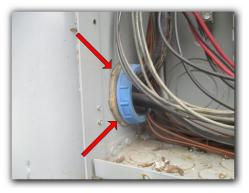
• There are no bonding jumpers across the flex connectors at the gas fired appliances.Inspector recommends bonding across the flexible gas lines at the gas appliances to reduce likelihood of lightning induced damage to the flex lines as the bonding capacity of the flex lines is unknown. This bonding may not be required by the Authority having Jurisdiction at the time of construction
