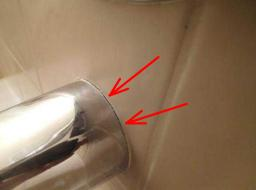
Ensure that all gaps at the escutcheons (where the plumbing penetrates the shower/tub enclosures) of the tub faucets, handles, and shower heads in the bathrooms are properly sealed (see photo).
