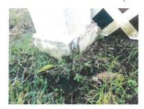
possible prior water contact. No moisture was detected using a surface moisture meter at the time of inspection.
