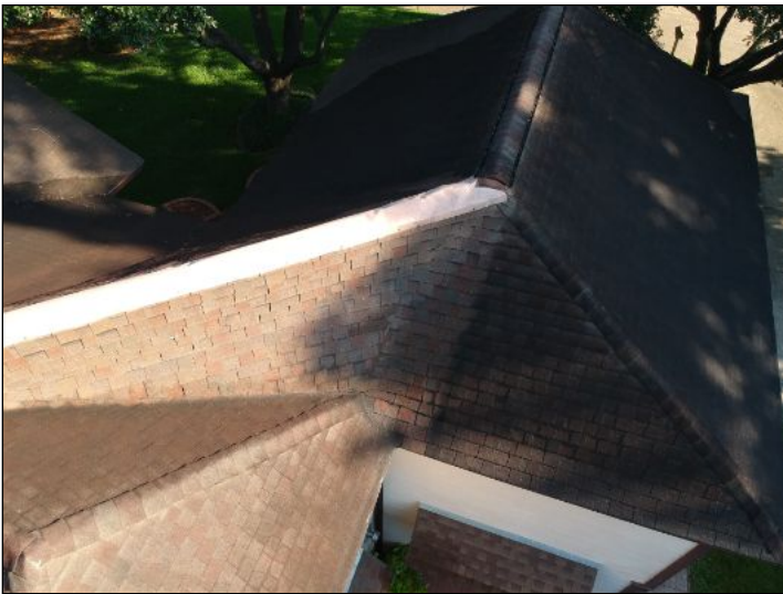
Overview of roof
