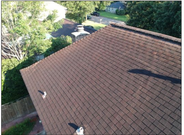
Overview of roof
