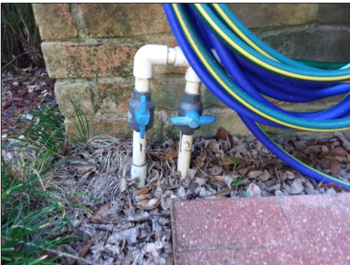
Zones 1 and 2 manual control located front/right, Zones 3 and 4 manual control located rear/right.
