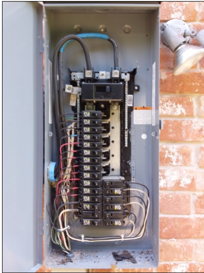
Overview of main electrical panel
