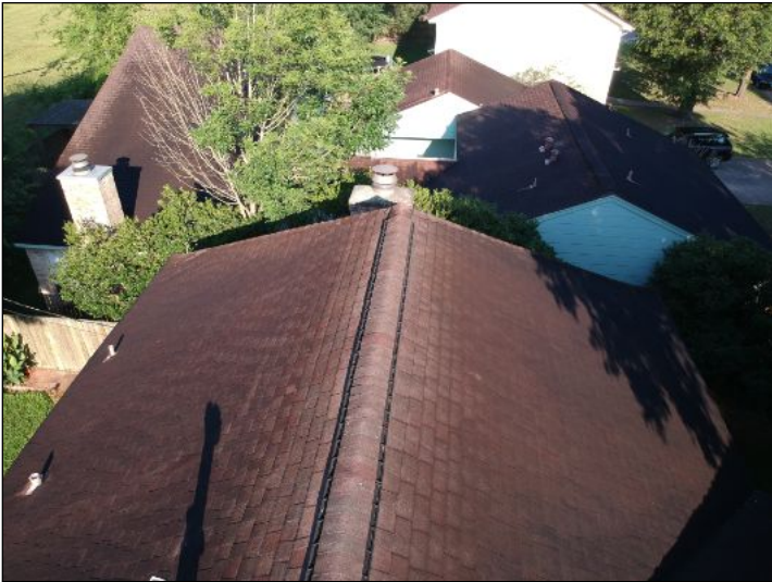
Overview of roof
