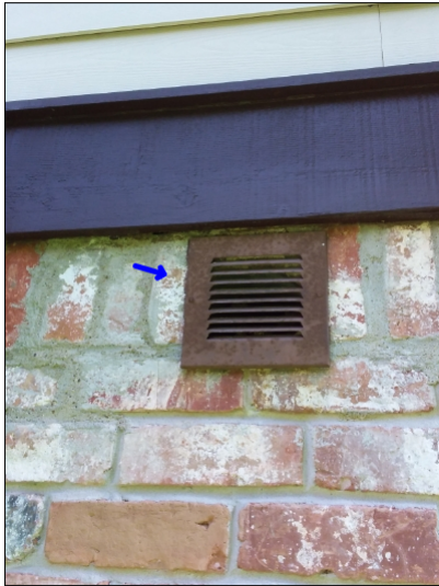
-Seal all vents at wall connection to help prevent water penetration into walls.
