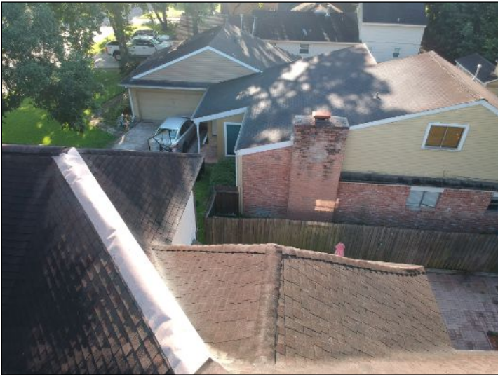
Overview of roof
