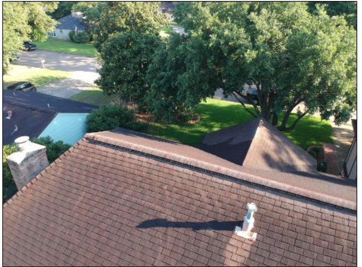
Overview of roof
