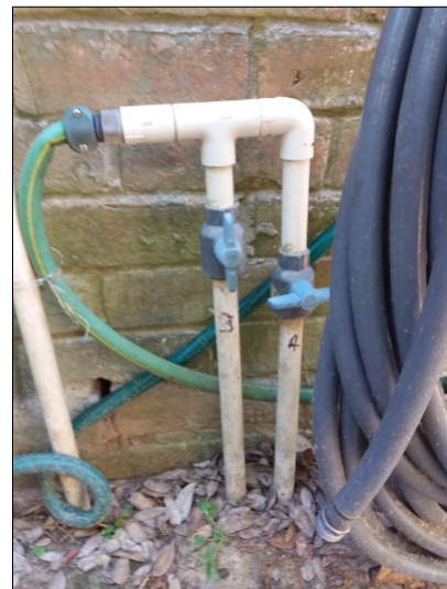
Zones 1 and 2 manual control located front/right, Zones 3 and 4 manual control located rear/right.
