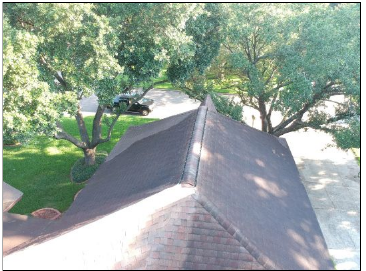
Overview of roof
