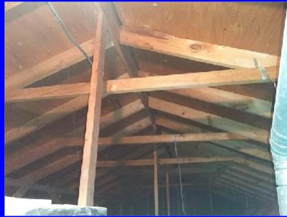
stick built with out radiant barrier
