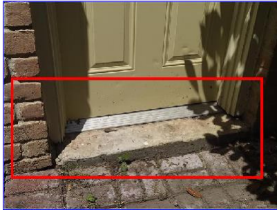
E. Item 16(Picture) left side garage door jamb
