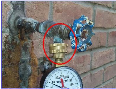
A. Item 2(Picture) all exterior faucets
