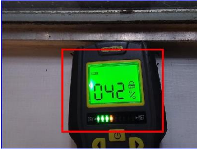
L. Item 6(Picture) living room window left side areas
