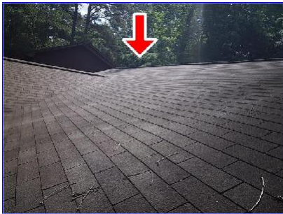
C. Item 8(Picture) multiple areas
