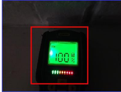
L. Item 7(Picture) living room window right side areas
