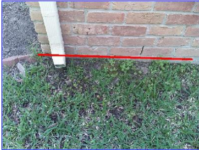
B. Item 3(Picture) right side of home
