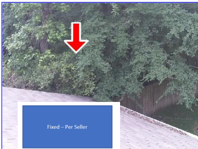
C. Item 1(Picture) rear of home areas
