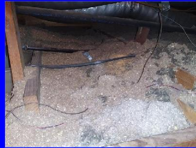
cellulose insulation 6 inches average
