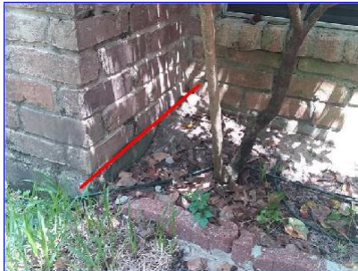
B. Item 6(Picture) rear of home areas
