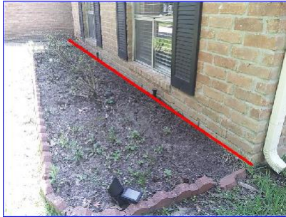
B. Item 4(Picture) front of home
