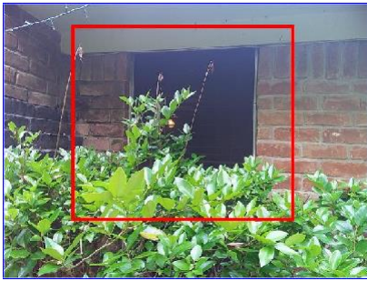
H. Item 1(Picture) rear of home areas
