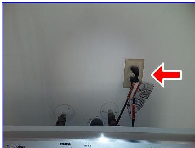
B. Item 2(Picture) washer dryer area
