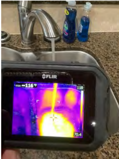
Hot water temperature reading on kitchen faucet at time of inspection was a normal range. Observational an informational purposes only
