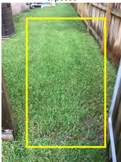
Ponding water noted on the right side of structure at time of inspection. Noted that it did rain hard today. No gutters noted on sides of house recommend adding gutters to deal with drainage
