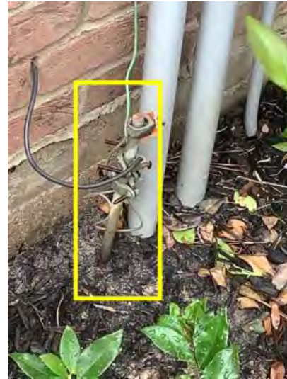
Grounding rod should be further in the ground noted. Recommend having a professional inspected correct.
