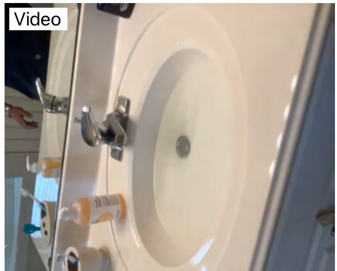
Master bathroom sinks were draining slowly at time of inspection recommend having a professional check for any obstructions or debris for optimal flow efficiency.
