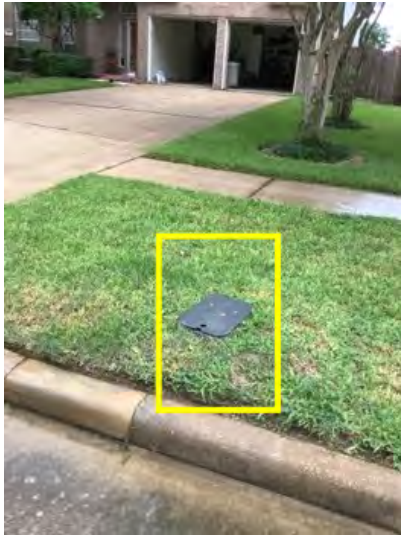
Main water meter located in front of property by sidewalk. Observational and informational purposes only.
