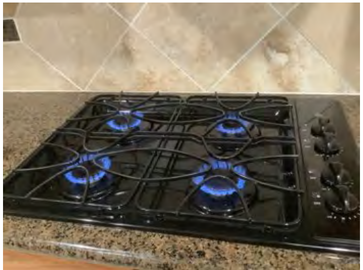
GE gas cooktop is working properly at time of inspection. Observational an informational purposes only
