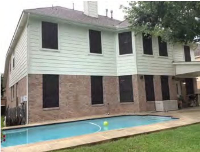
Back view of structure at time of inspection. Observational an informational purposes
