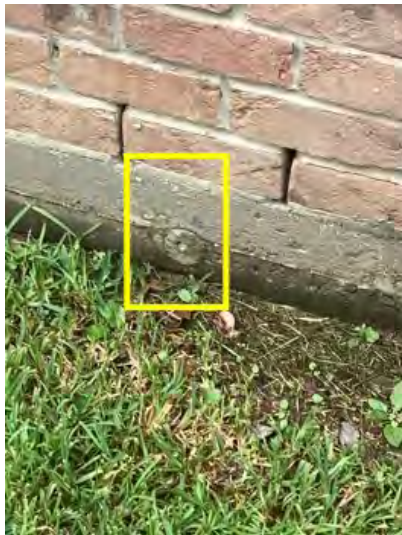
Post tension foundation penetrations noted at time of inspection. Observational an informational purposes only.
