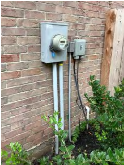
Electrical grounding rod meter and underground service noted at time of inspection. Meter located on the right side of house at time of inspectio
