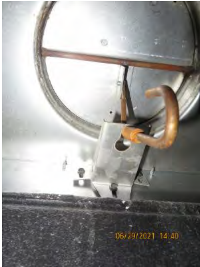
View of fireplace damper noted. Observational an informational purpose only.
