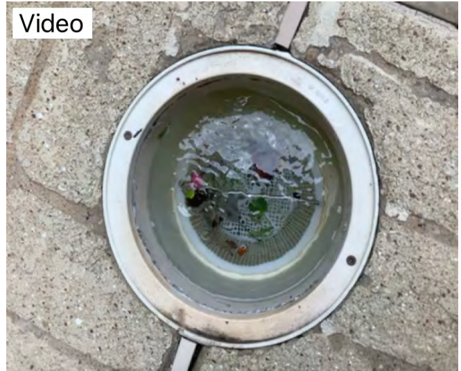
Video of skimmer basket clean and flow working properly at time of inspection. Observational an informational purposes only
