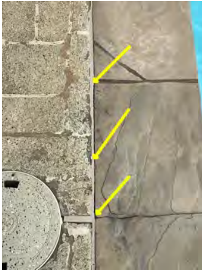
All caulking around pool between decking and coping should be sealed properly conducive to moisture intrusion, damage, expansion and contraction. Recommend having a professional inspecting correct.
