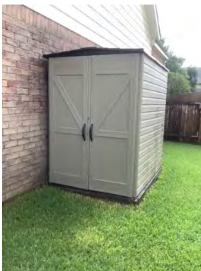
Small plastic shed noted on left side of property at time of inspection. Unit was not inspected just observed.
