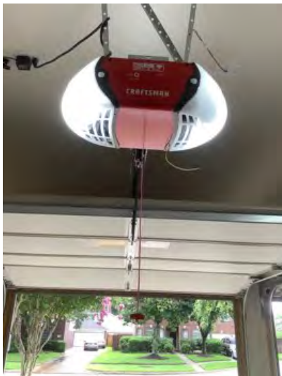
Craftsman automatic garage door opener noted at time of inspection. Observational purposes only
