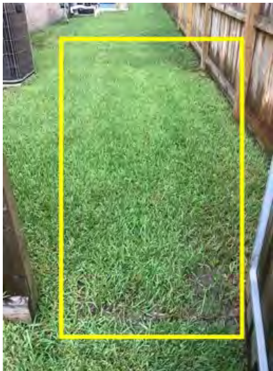
Ponding water noted on the right side of structure at time of inspection. Noted that it did rain hard today. No gutters noted on sides of house recommend adding gutters to deal with drainage
