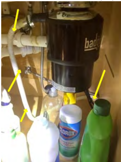
Dishwasher high Loop drain noted at time of inspection should be secured the top of the cabinet in order to prevent anti-siphon and backflow. Recommend having a professional inspection correct
