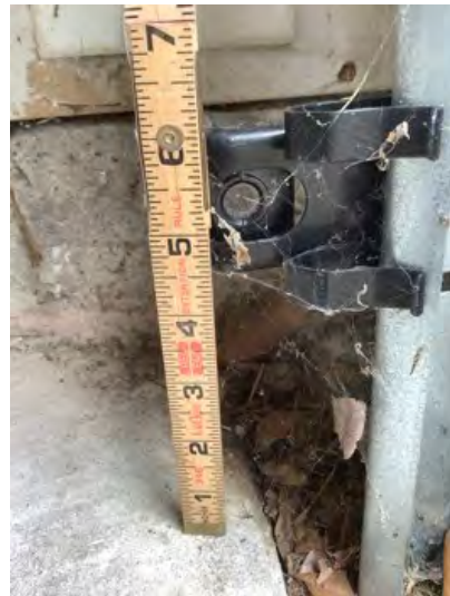
Garage door electric back up sensors one or approximate range of 6 inches noted. Observational and informational purposes only
