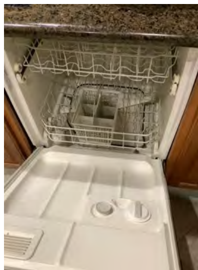
Interior view of dishwasher noted at time of inspection. Observational an informational purposes only.
