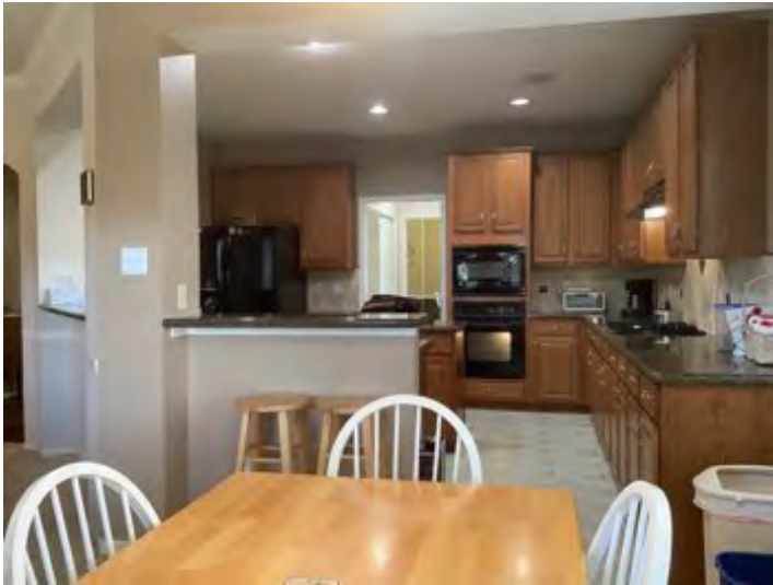
Kitchen area noted at time of inspection. Observational an informational purposes only.
