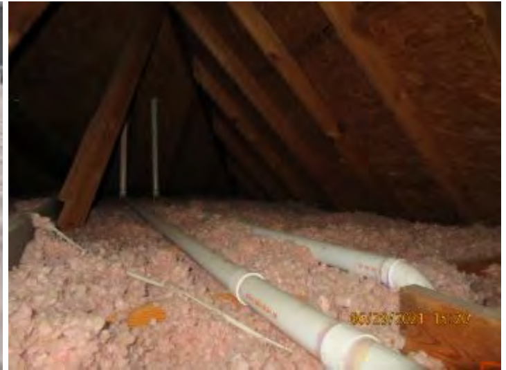
Limited access area in attic noted. Observational an informational purpose only.
