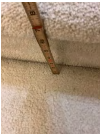
Stairs rise measurement was a normal range at time of inspection. Observational an informational of
