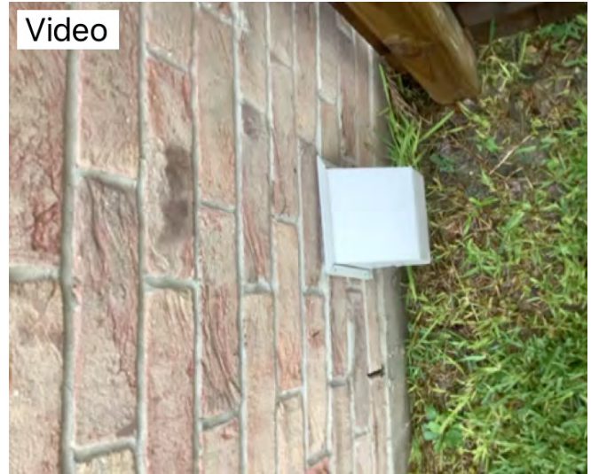
Dryer vent located on the left exterior of property noted not secured see you and talk properly to structure. Conducive to moisture intrusion, damage and potential WDO. Recommend having a professional inspect and correct
