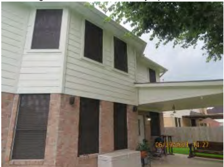
Back patio noted. Observational an informational purpose only.
