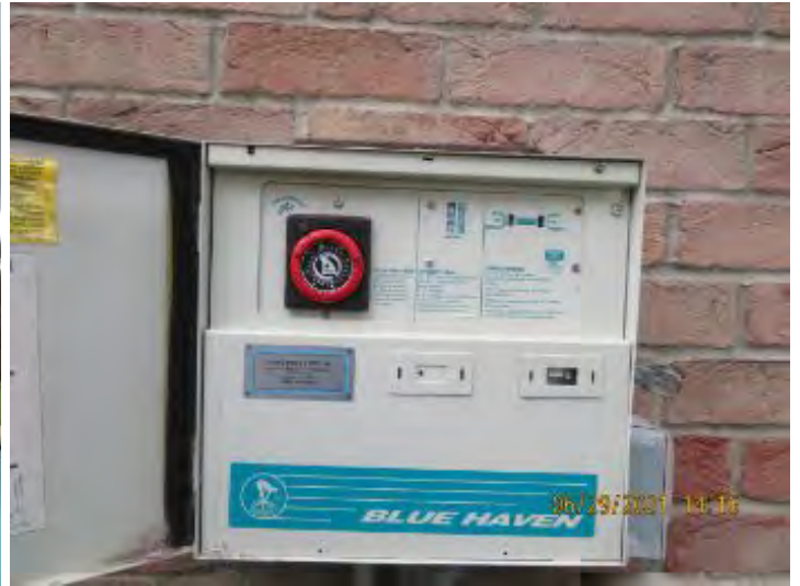
Interior view of panel noted. Observational an informational purpose only.
