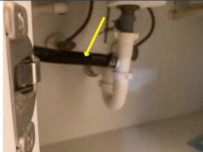
Main condensation drain noted under sink and guest bathroom at time of inspection. Observational an informational
