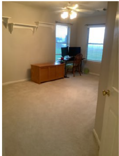
Second-floor bedroom left side noted at time of inspection. Observational an informational purposes only
