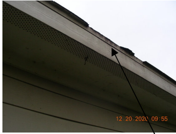
Examples of damaged shingles
