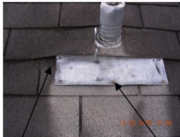
Examples exposed nail/bolt heads and raised roof jack flanges
