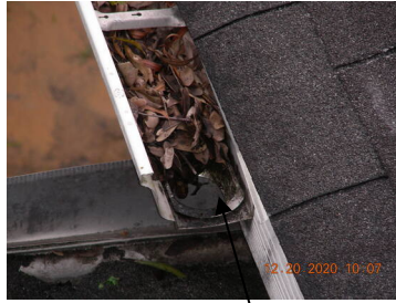
Example of damaged gutters and gutters filled with debris
