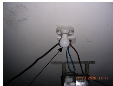
Exposed light bulbs in garages need protection
