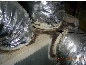
Mildew staining on A/C air boxes in attic on both units
