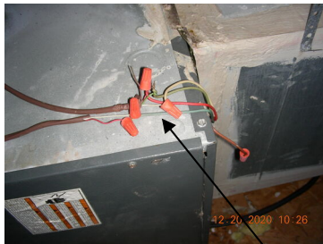
Exposed, unprotected wire splices on both A/C units in the attic
