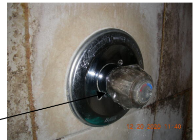
Unit B primary bathtub faucet handle has reversed water output when the respective temperatures are selected
