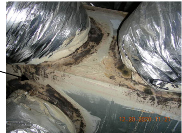
Mildew staining on A/C air boxes in attic on both units
