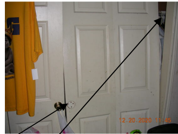
Detached hinge on bedroom entry door in unit B
