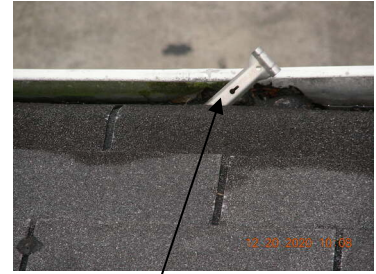
Example of detached gutter bracket
