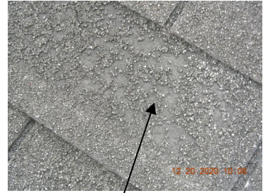
Examples of delaminated shingles
