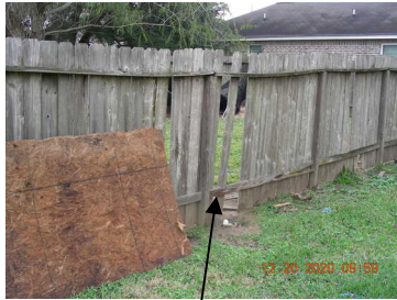
Examples of damaged fence boards and fence gate without latch on inside of gate
