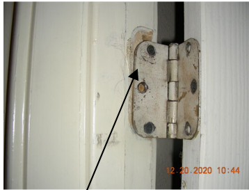
Detached hinge on bedroom entry door in unit B
