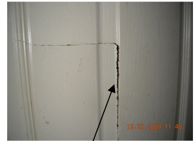
Damaged entry door to primary bedroom in unit A
