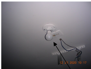
Exposed light bulbs in garages need protection
