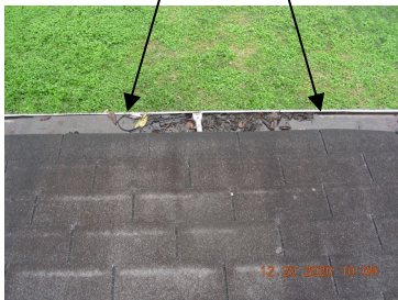
Example of sagging and leaking gutter and gutter holding water
