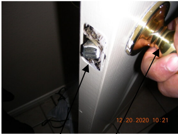
Laundry room door knob does not fully turn in unit B
