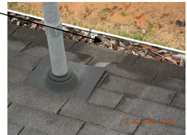
Example of detached gutter bracket
