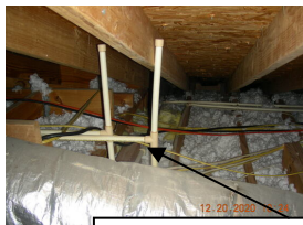
Examples of exposed pipes and inadequate amounts of insulation in the attic
