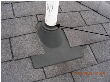
Examples exposed nail/bolt heads and raised roof jack flanges
