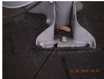
Examples exposed nail/bolt heads and raised roof jack flanges
