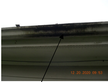
Example of sagging and leaking gutter and gutter holding water
