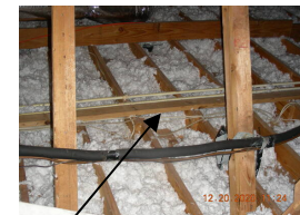
Examples of exposed pipes and inadequate amounts of insulation in the attic
