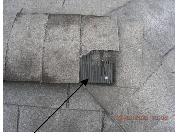
Examples of damaged shingles
