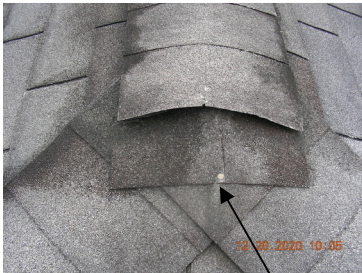
Examples exposed nail/bolt heads and raised roof jack flanges
