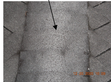
Examples of delaminated shingles
