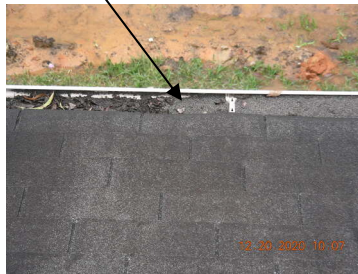
Example of damaged gutters and gutters filled with debris
